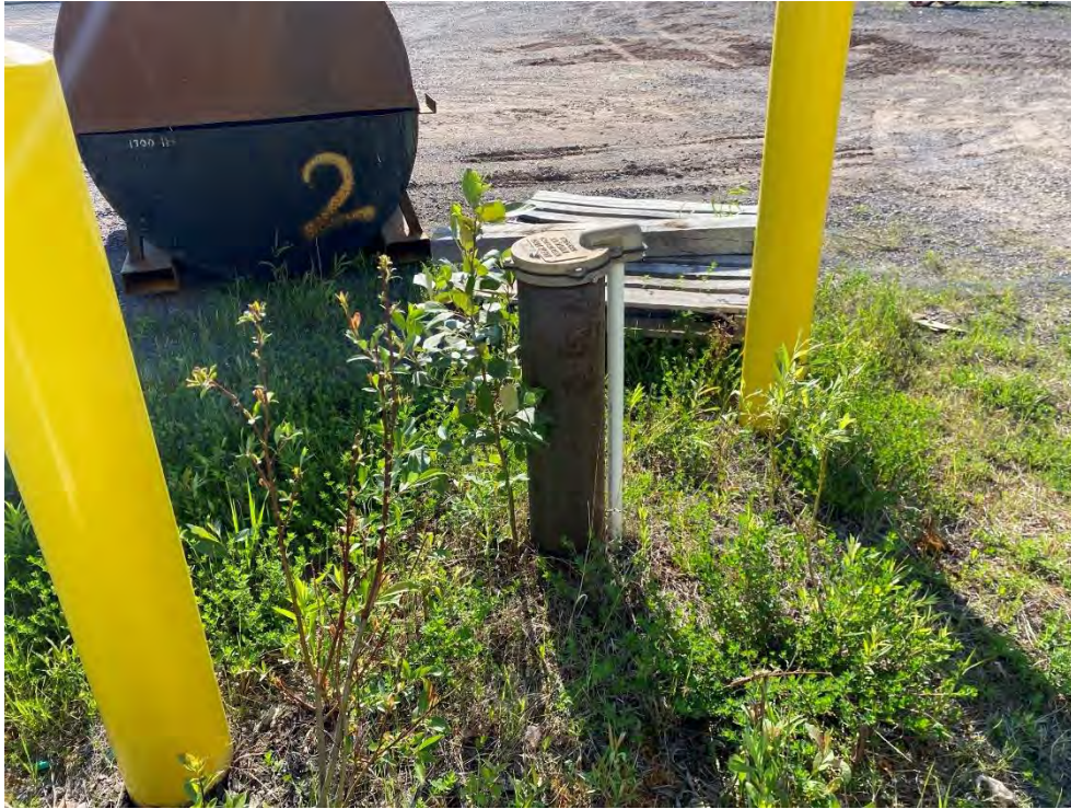
Photo 1: Private Well PW-2, photo facing west.
