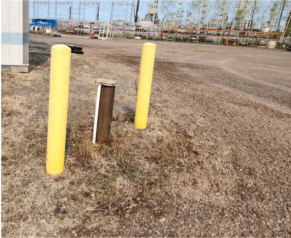
Photo 1: Private Well PW-2, photo facing northwest. (May 17, 2023)
