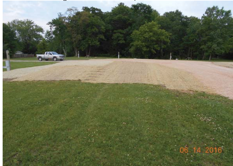
Phot #18: Facing east. Finished cap.
