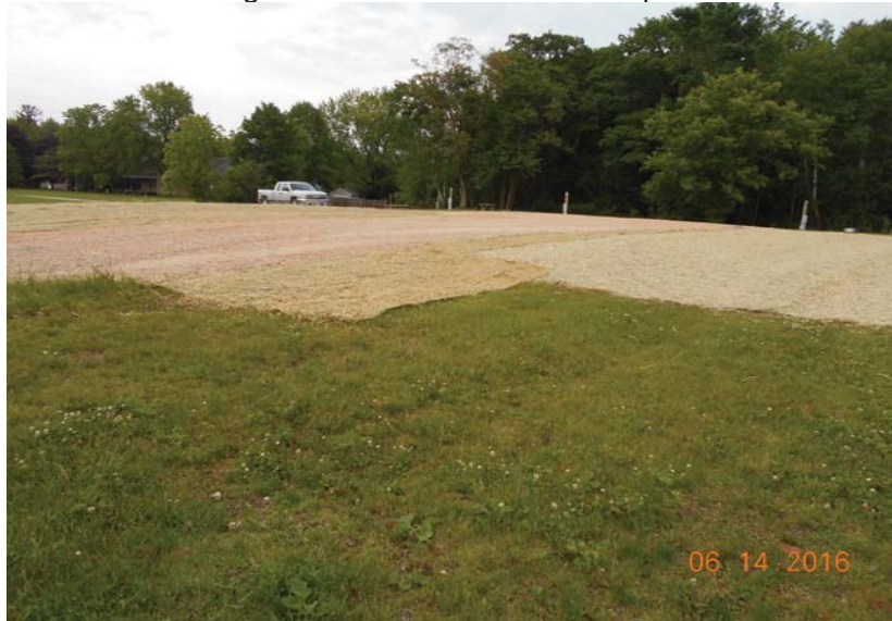
Photo #17: Facing east/northeast. Finished cap.
