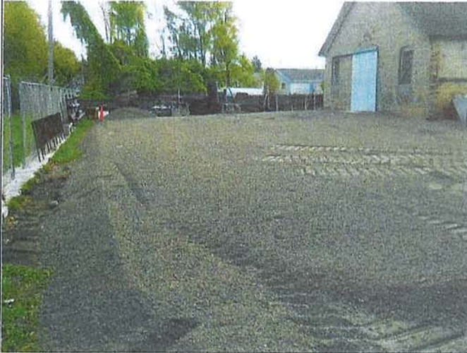
Title: Photo #1: Area of cap to be maintained (looking east)
