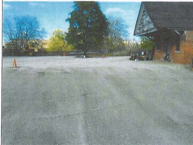
Title: Photo #1: Area of cap to be maintained (looking north)
