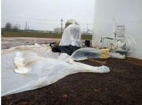
Photo 1: Plastic sheeting and absorbent boom installed to prevent contaminant migration (May 20, 2013).
