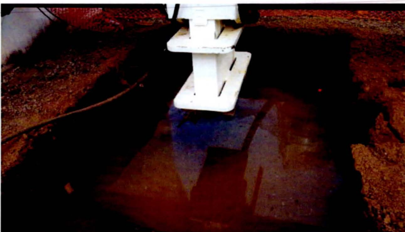
Photo 2: Tank 11 valve maintenance excavation with trace amounts of sheen on water surface. 7/8/2014
