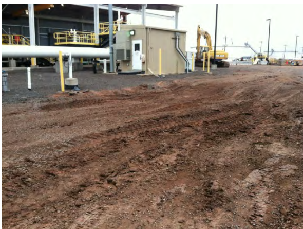
Photo 3: Remedial excavation at the release location (facing north).
