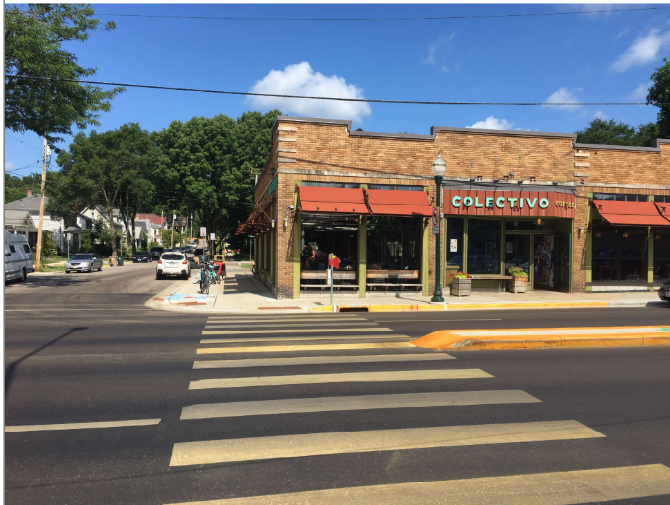
Title: Building, Looking Northwest - August 8, 2019.
