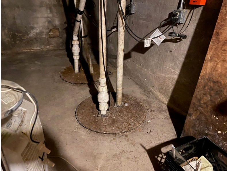
11. Sumps located near East U-Tube location, facing north.
