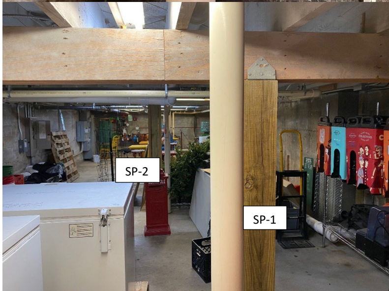
6. Two floor penetrations, SP-1 and SP-2 (West U-Tube location), facing southeast.
