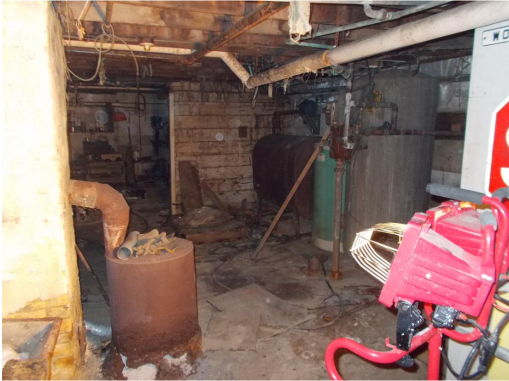
5) View of the basement and general location of SB/TW-7
