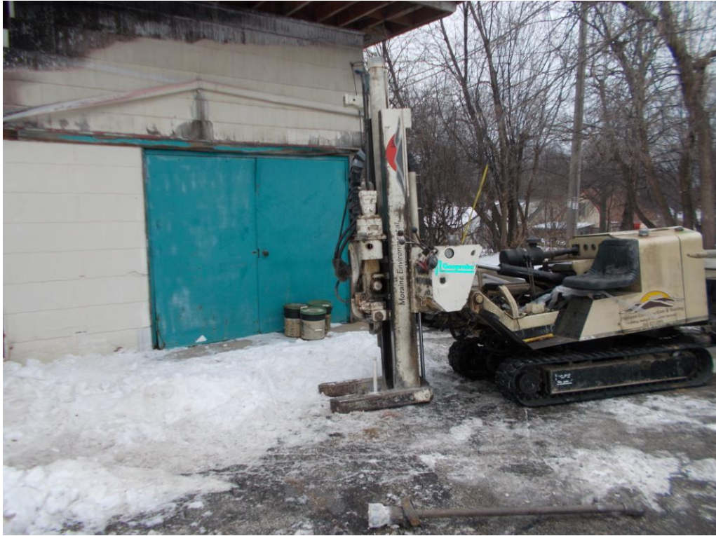
3) Location of SB/TW-5 being completed with temporary monitoring well
