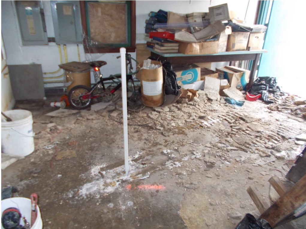
1) SB/TW-1 completed with temporary monitoring well
