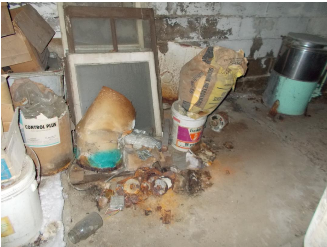
8) View of the basement and general location of SB/TW-3
