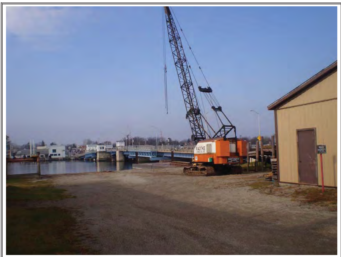
Site # 9 Radtke Contractors, Inc., 15 and 21 E. Main Street, View west from west side of 1 st Avenue
