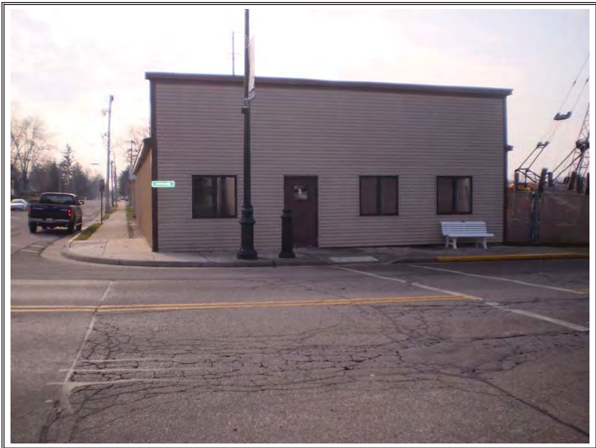
Site # 9 Radtke Contractors, Inc., 15 and 21 E. Main Street, View south from north side of Main Street
