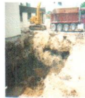
CONTAMINATED SOIL EXCAVATIONS
