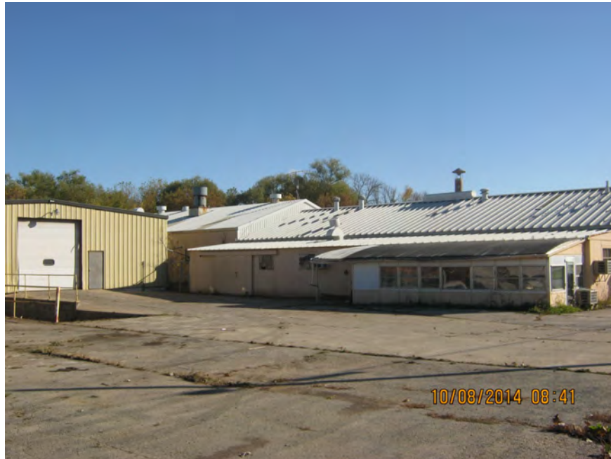
Photo 1: View of the 420 East Main subject property parcel from the southwest.
