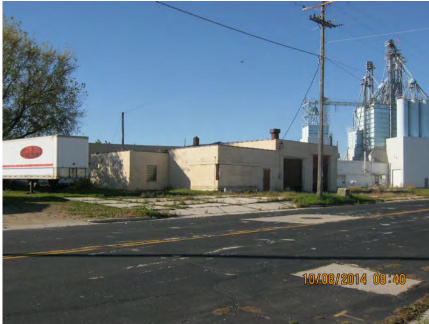
Photo 3: View of 415 East Main Street subject property parcel from the northeast.
