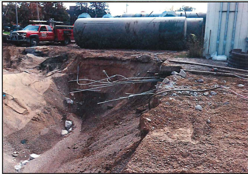
Facing South - Tanks Out - Former Tank Bed
