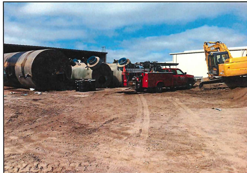
Four (4) USTs Removed From Site
