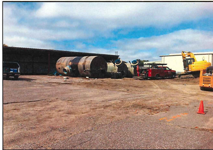
Facing Northwest at Tank Bed - Tanks Excavated
