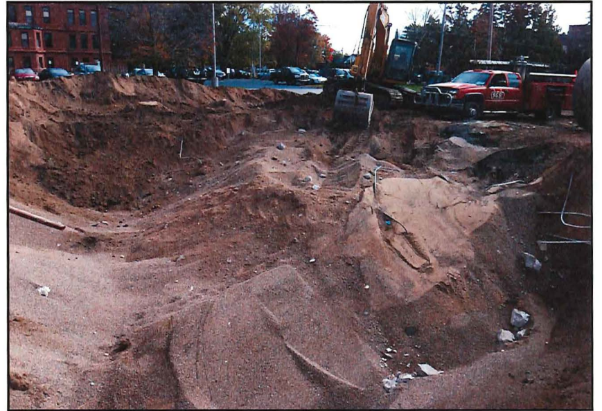
Exposed Tank Bed
