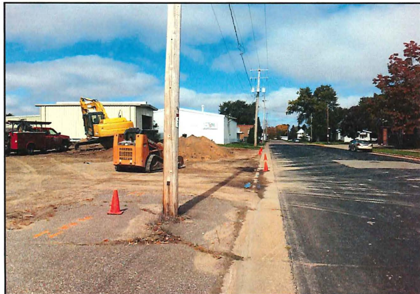
Facing North - Looking Up Edison Street
