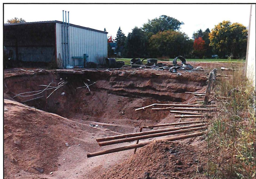
Exposed Former Tank Bed
