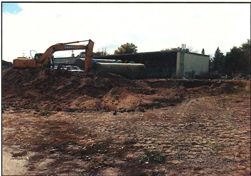
Facing Southwest at Tank Bed
