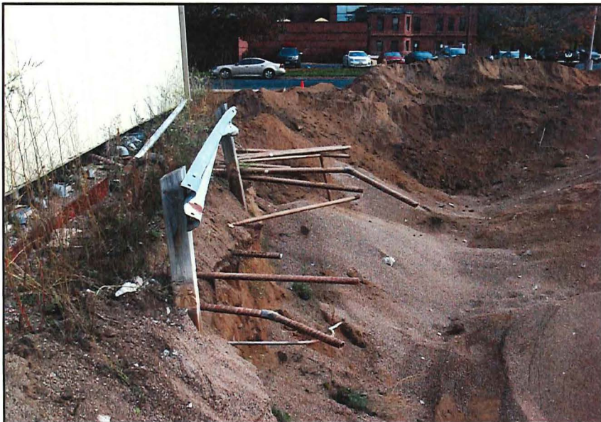
Exposed Tank Bed
