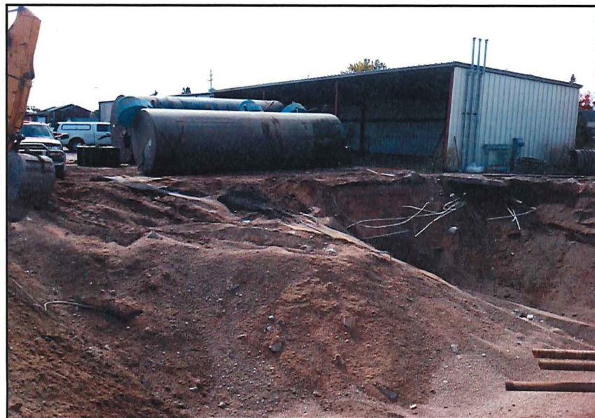
Exposed Former Tank Bed
