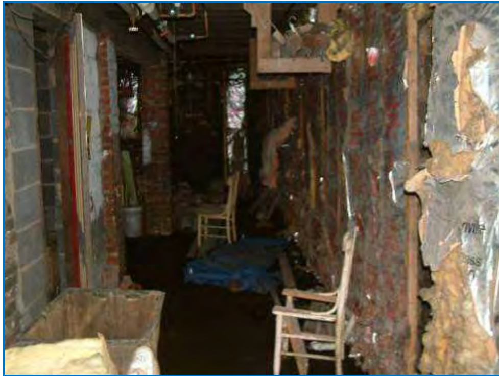
Photo #11 Basement hall, looking east toward Stevens Street.
