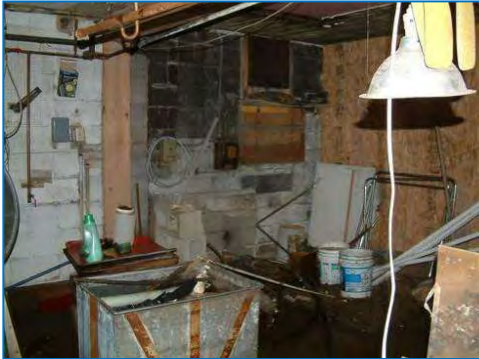
Photo #41 In the shop, near the boiler room. The earthen opening in the concrete cited as a REC is located under the white 5-gallon pails in the background.
