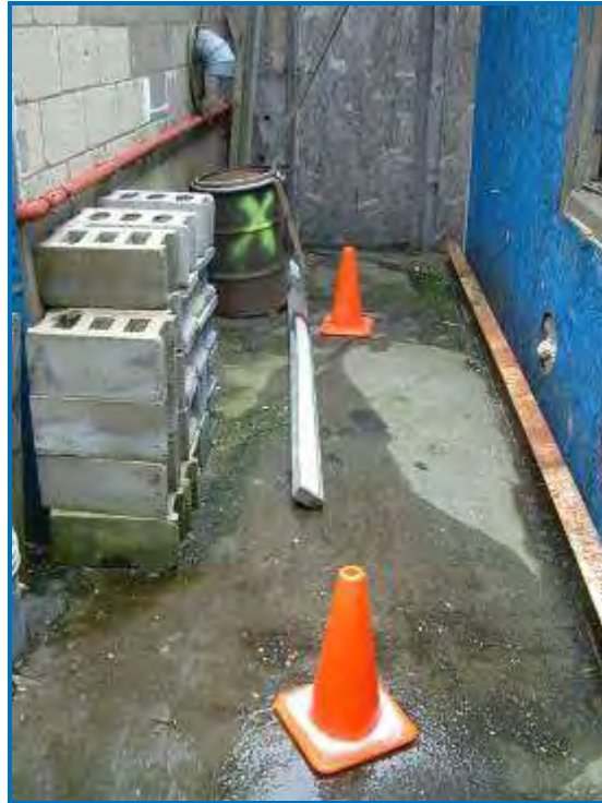
Photo #19 Outdoor storage area. The two cones represent former USTs Nos. 6 (foreground) and 7 (background) on Figure 4.
