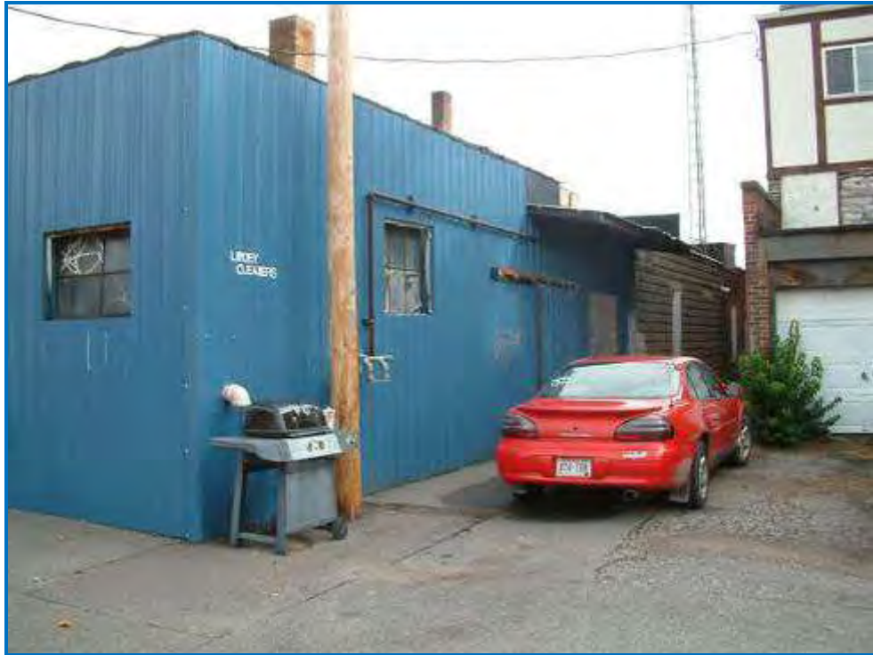
Photo #5 Looking at the southwest corner of the Lindy Cleaners building.
