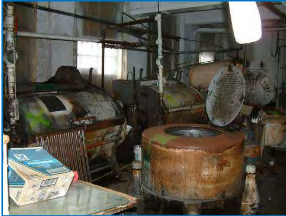
Photo #29 Another view of the dry cleaning area, looking northwest. Yellow paint denotes machines with visible solvent in them.
