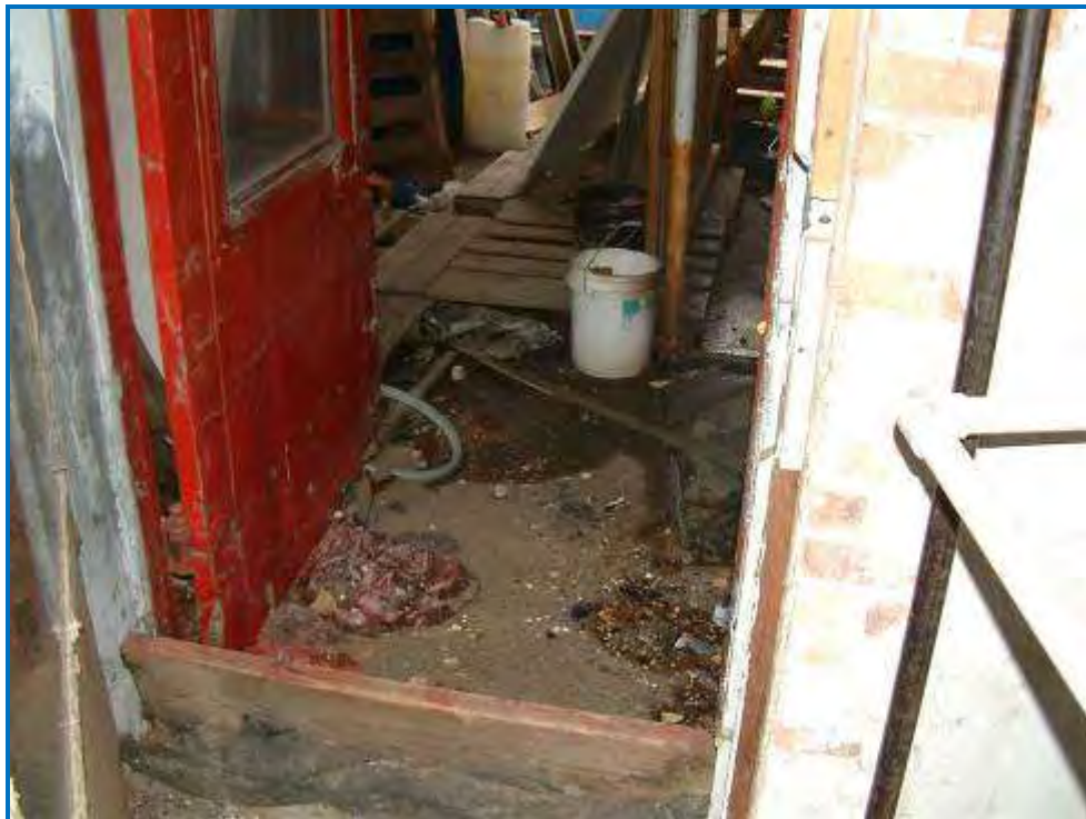
Photo #18 Entrance to the outdoor storage area.
