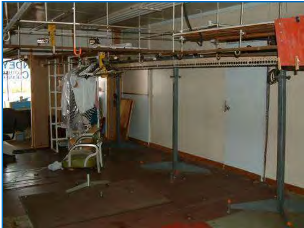
Photo #42 General view of the finished laundry area, looking east toward Stevens Street.
