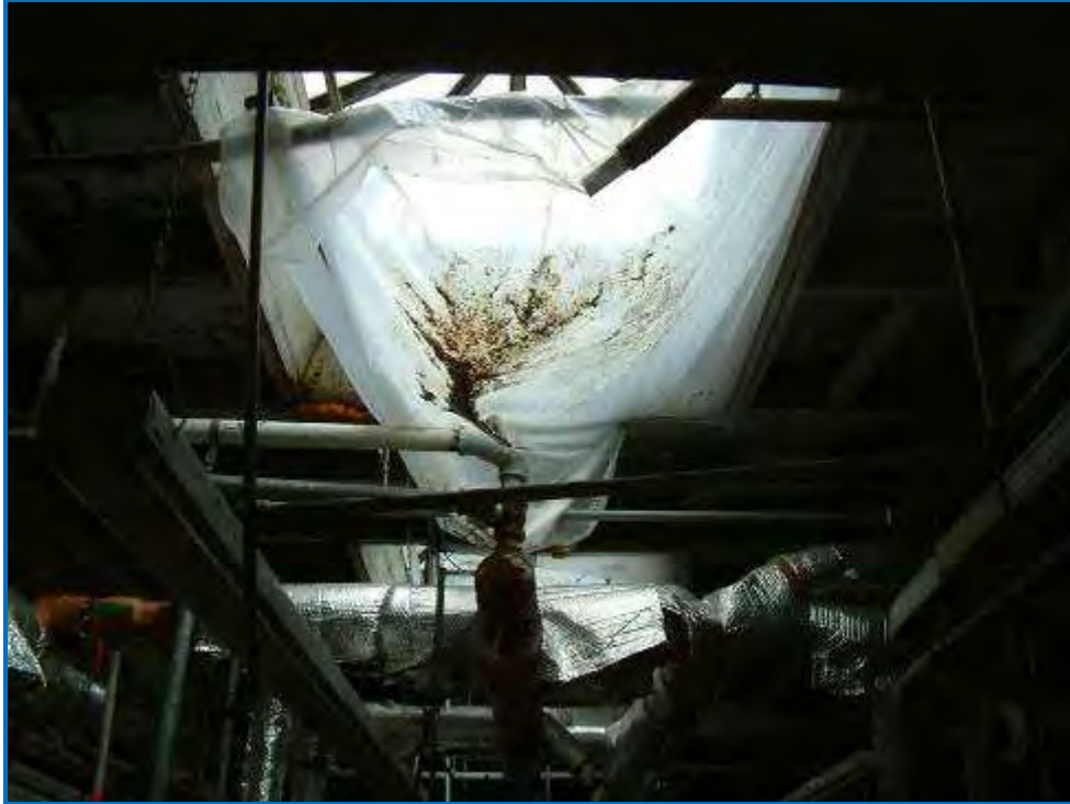
Photo #35 The roof in the steam laundry is in rough shape. The rain falls on the asbestos and causes it to disintegrate.
