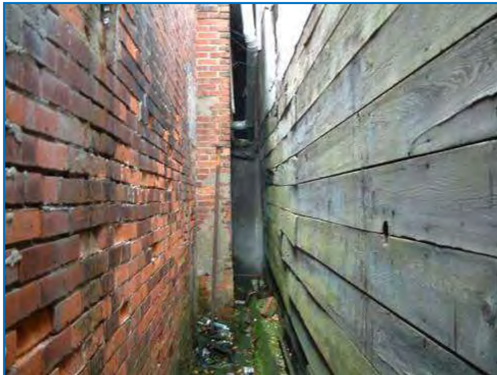
Photo #4 Between the two buildings on the Property . Note what looks like a UST vent about 5 feet high against the brick wall in the back. No known UST that this would be connected to.
