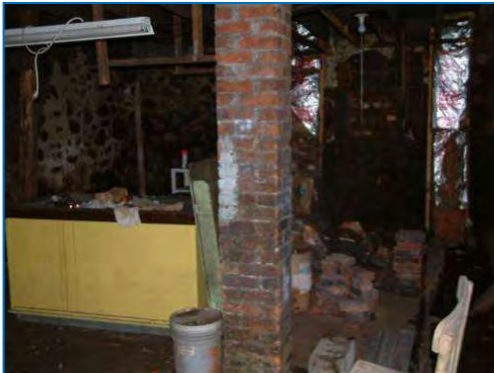
Photo #12 Basement front room, along Stevens Street in the background.
