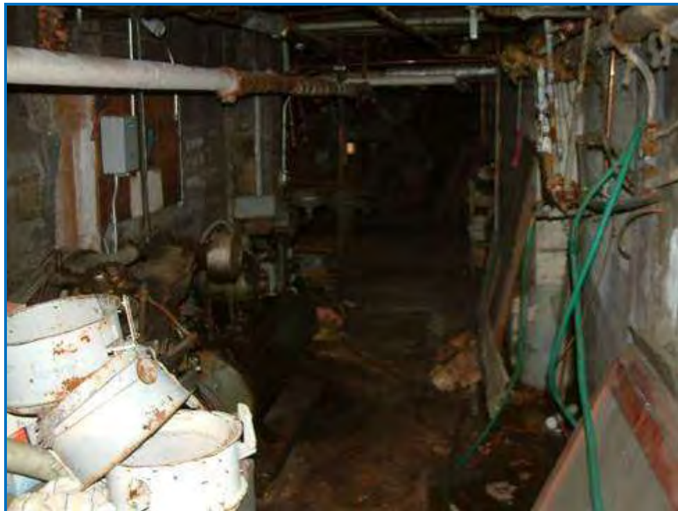
Photo #8 Basement, looking east. Lots of miscellaneous stuff in the basement.
