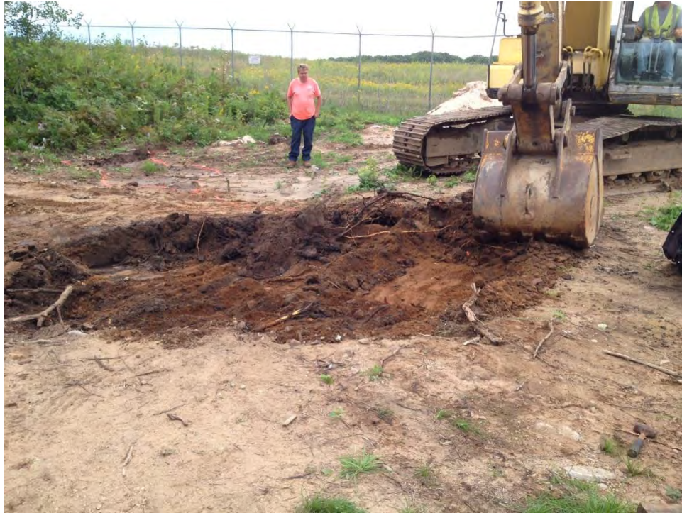
Photo #7 Excavating in the primary spill area.
