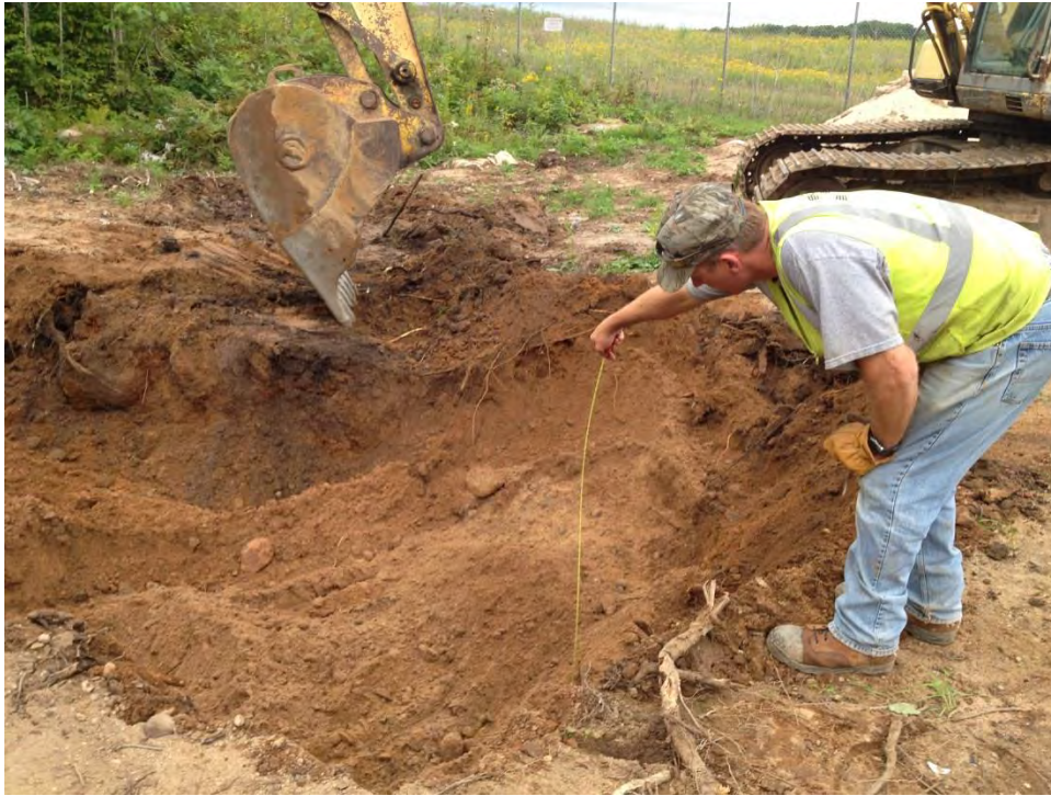
Photo #11 Completed excavation in the primary spill area at 4.5 feet.
