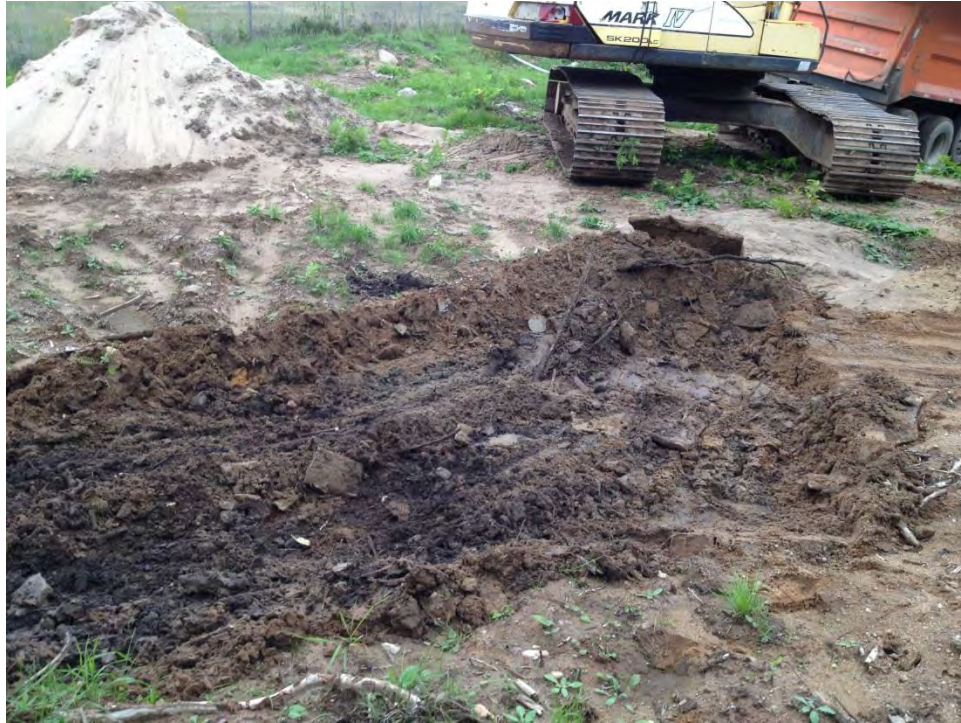
Photo #9 Excavating in the secondary spill area.
