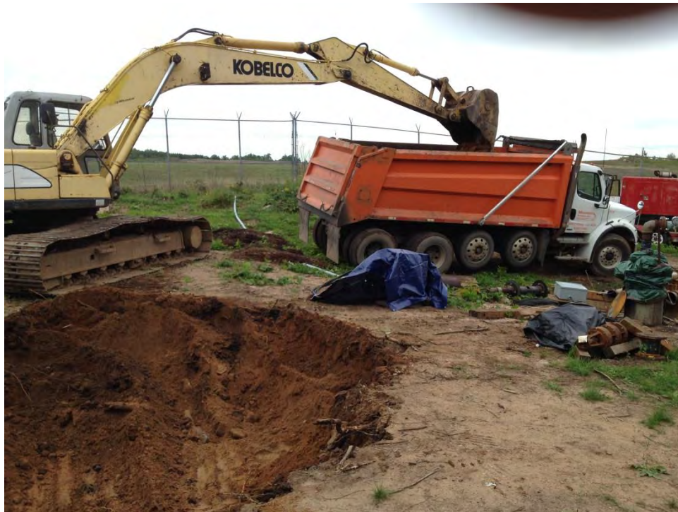
Photo #8 Excavating in the primary spill area.
