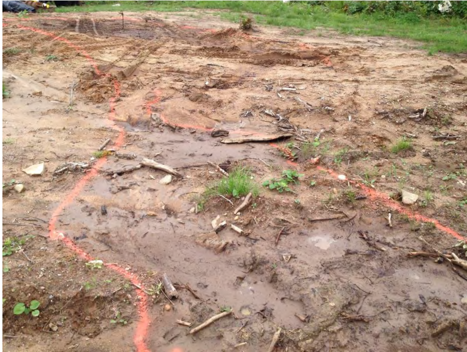
Photo #5 Secondary spill area in the foreground. Primary spill area in the background. Looking east.
