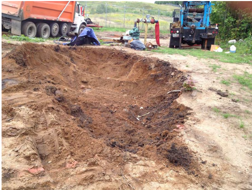
Photo #10 Completed excavation in the primary spill area at 4.5 feet.
