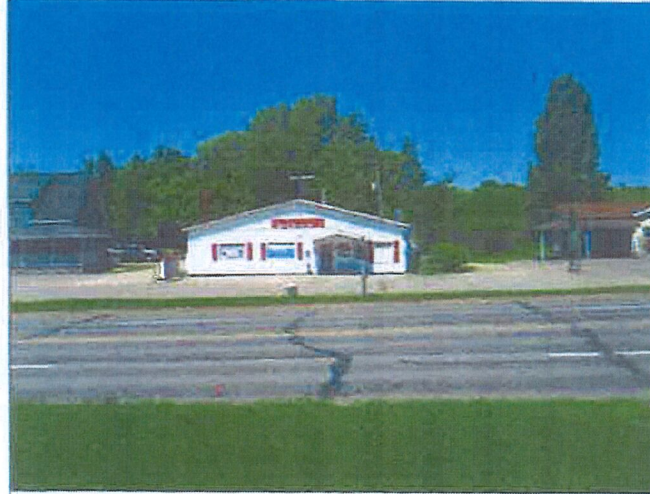
Title: Photo 2#: Area of cap to be maintained (looking northwest)
