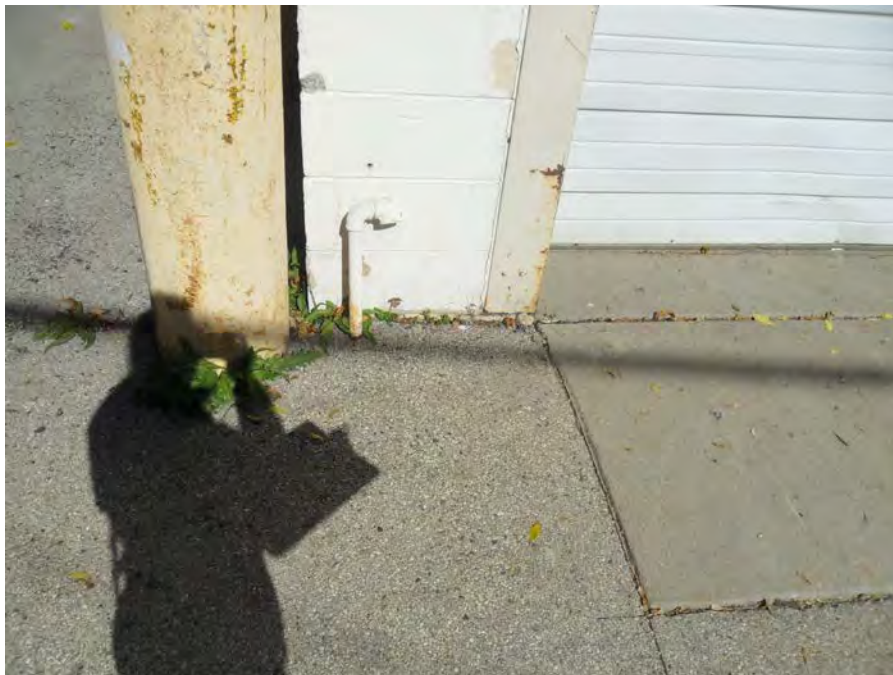
Photo 6: View of pipe outside the Ace Hardware unit.
