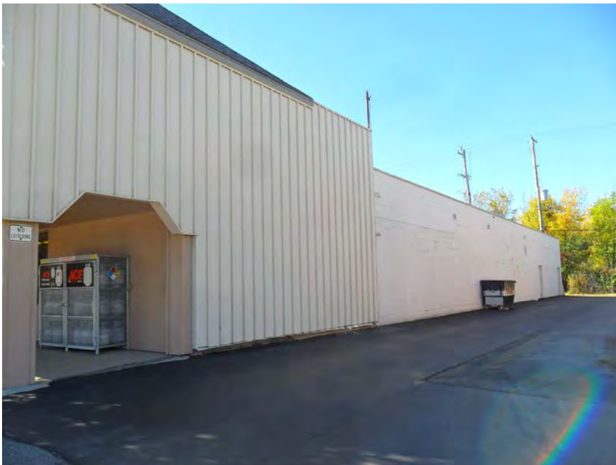
Photo 2: View of the north side of the building on the Subject Property, looking west.
