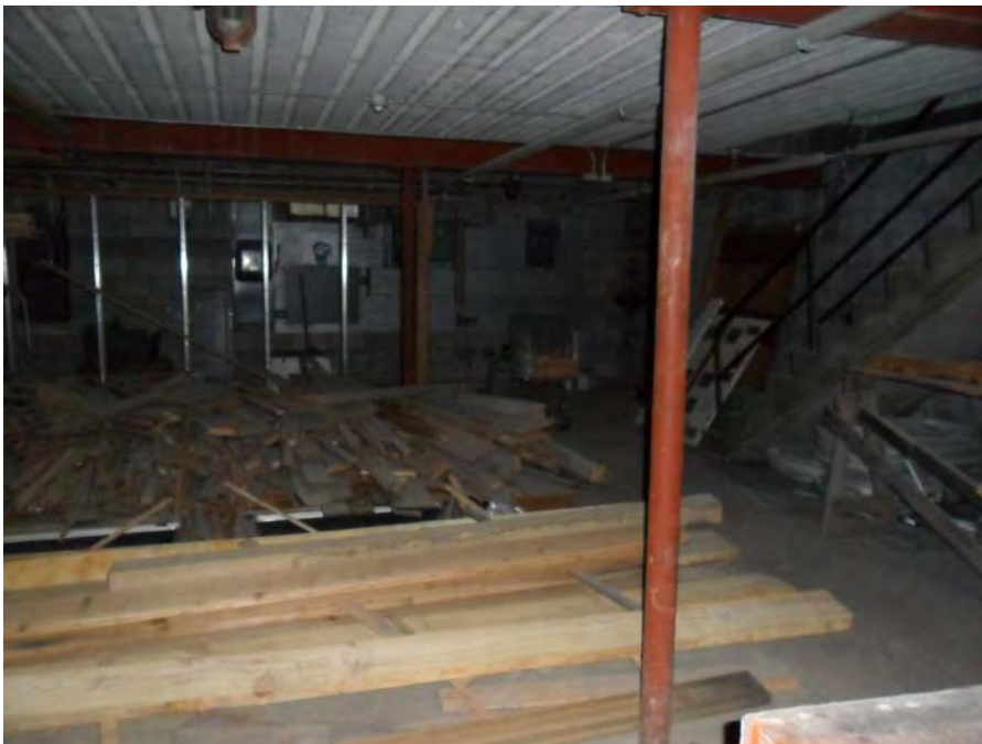
Photo 4: View of the basement in the Ace Hardware unit.
