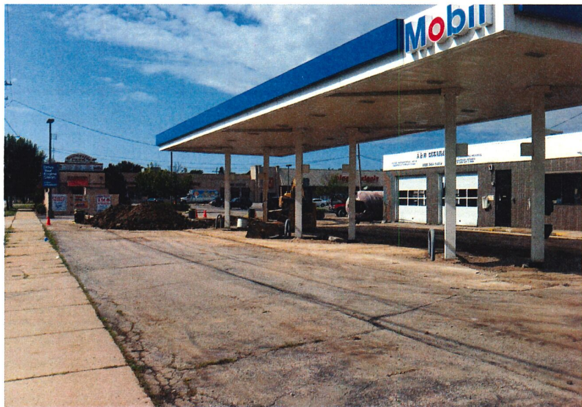
Facing Southwest at Pump Island
