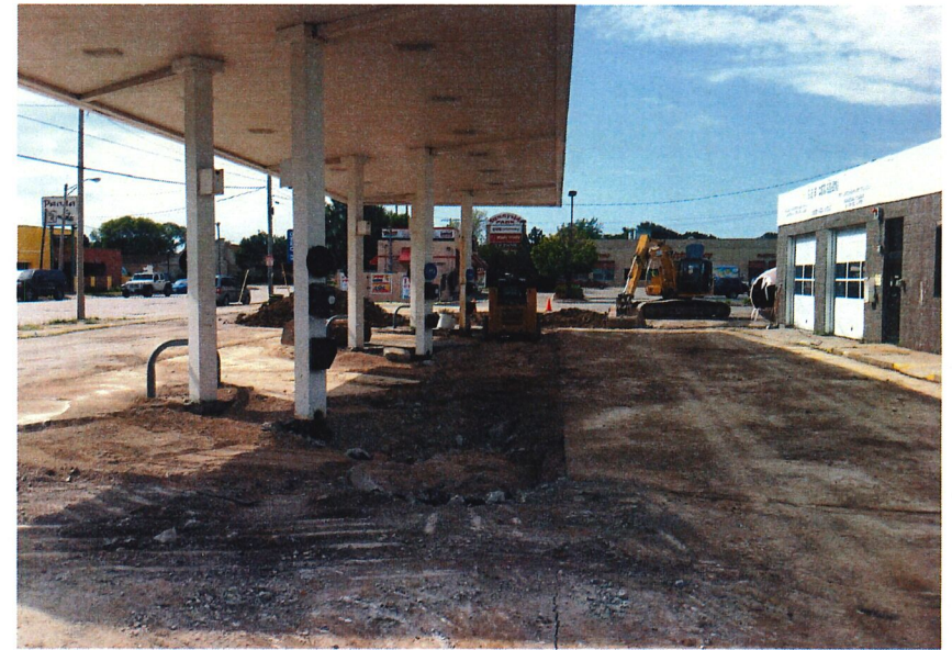
Facing South - Piping Trench
