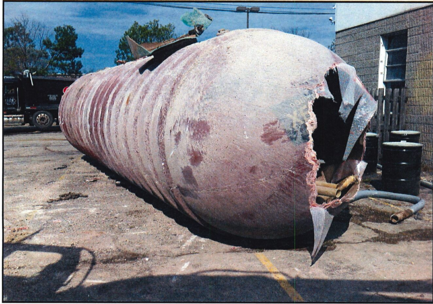
12,000 gallon UST Removed From Site
