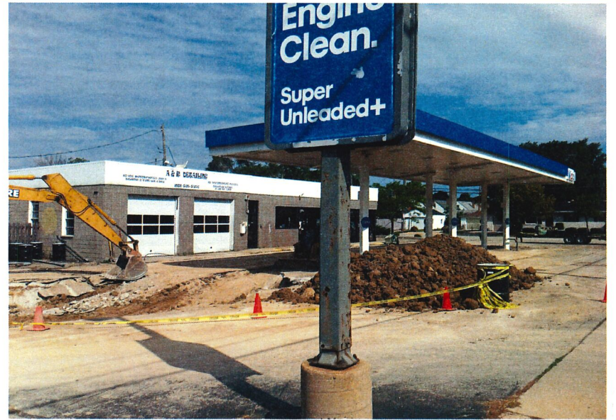
Tank Bed - South of Pump Island
