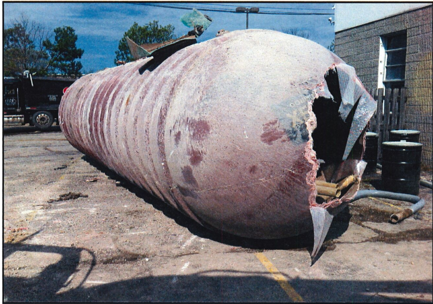
12,000 gallon UST Removed From Site
