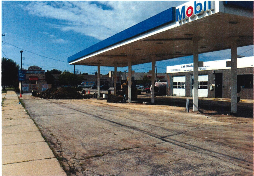
Facing Southwest at Pump Island
