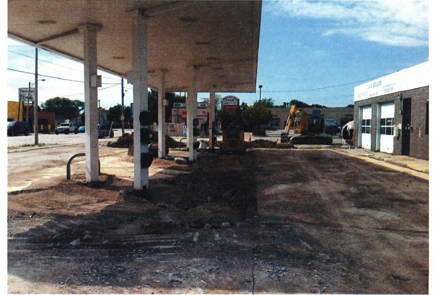
Facing South - Piping Trench
