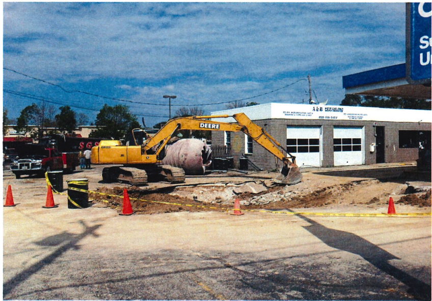
Facig Northwest at U.S. Petroleum Station Tank Bed
