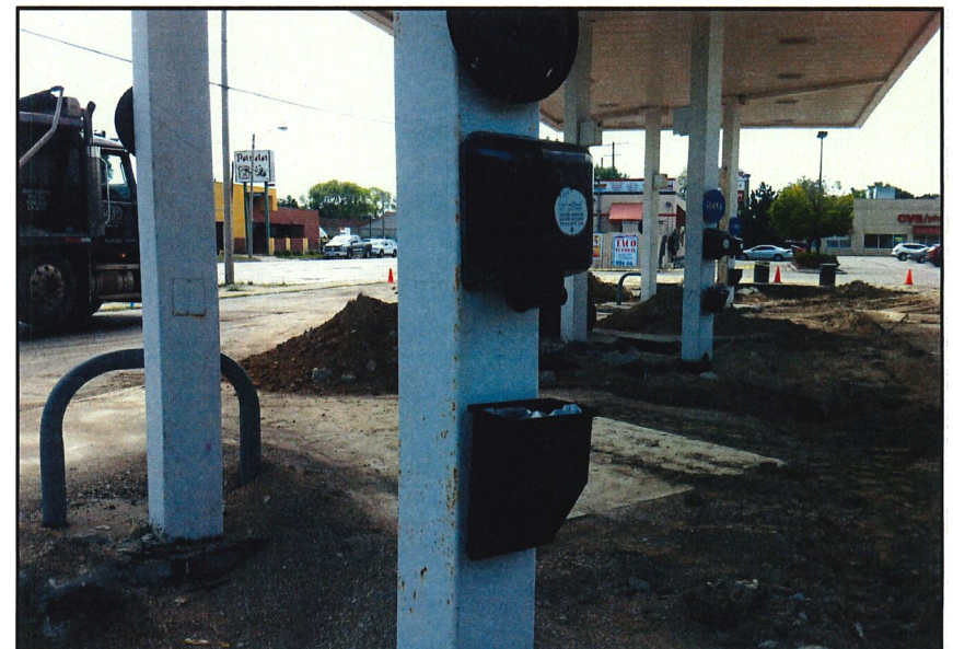
Dispenser Island - Piping Sampling
