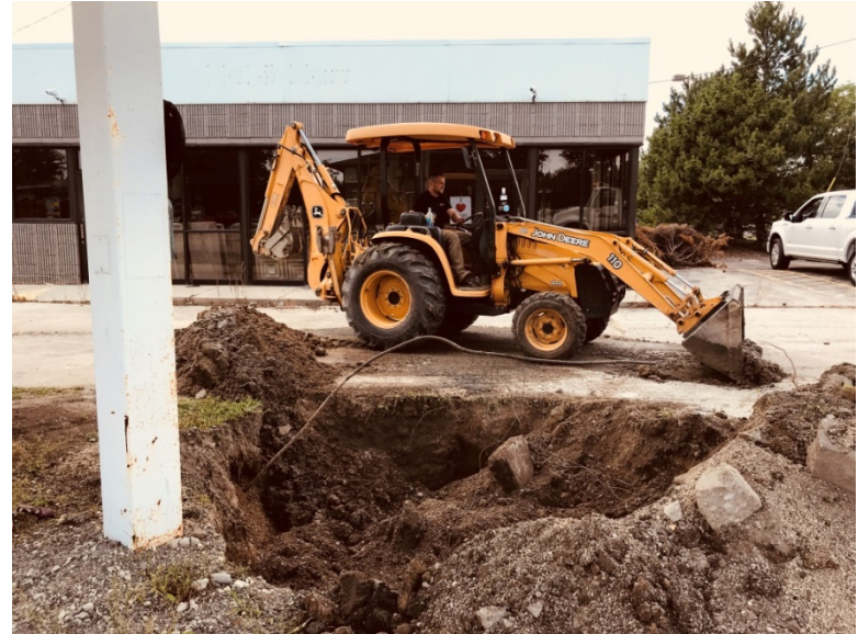
Clean fill to right, Bio-pile contaminated soil at far left
