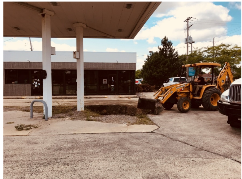
Excavation trench backfilled
