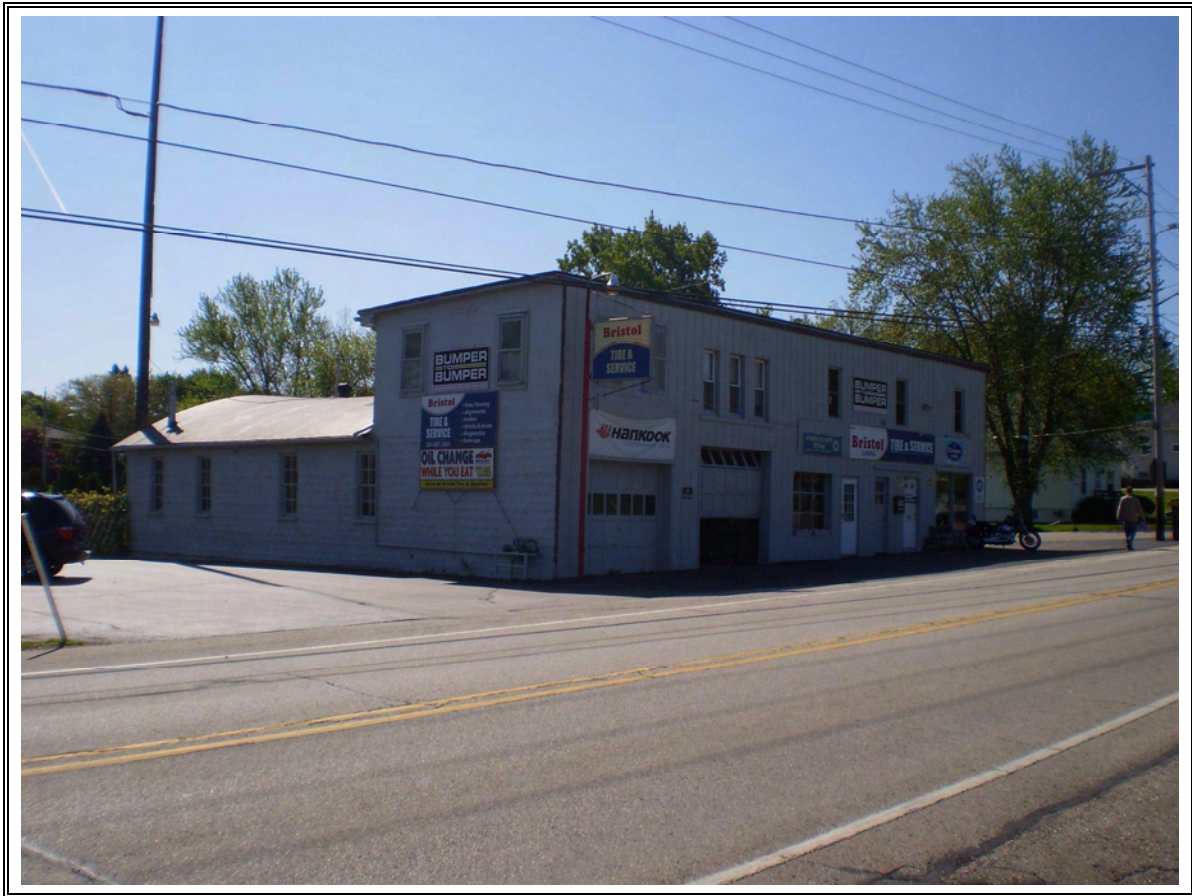
Site #2: Bristol Garage, 8335 200 th Avenue. View southeast from west side of USH 45
