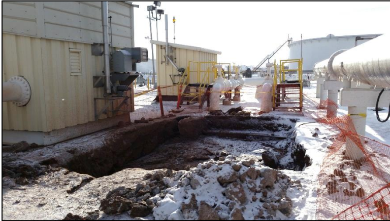
Photo 1: Line 1 Skid excavation. Photo facing southwest on November 19, 2014.
