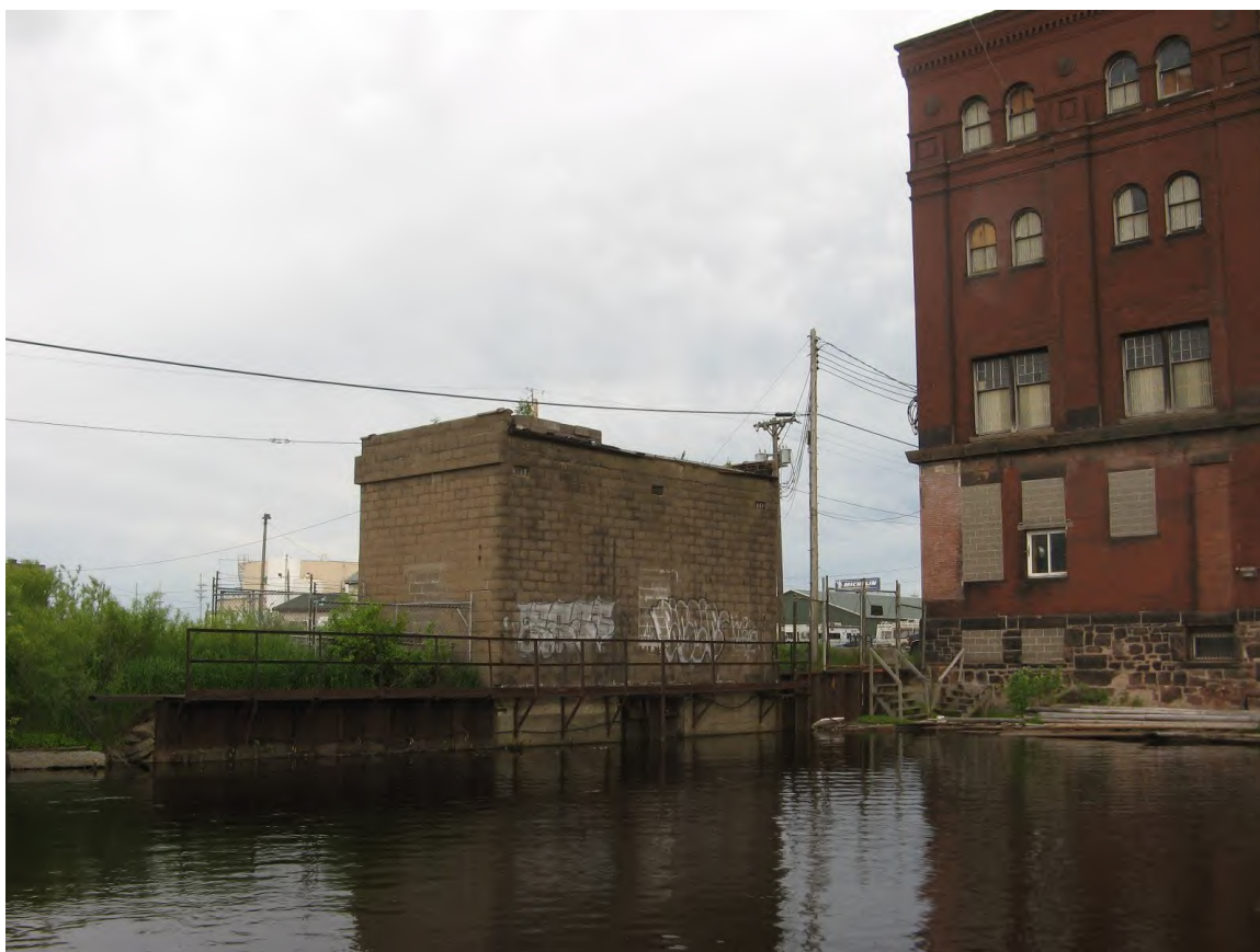
End of warehouse and possible old intake structure in Hughitt Slip
