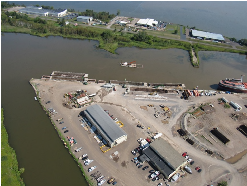
Figure 3-1. Support Area Aerial Photograph (provided by USACE); additional aerial photographs can be found on the project SharePoint f .
