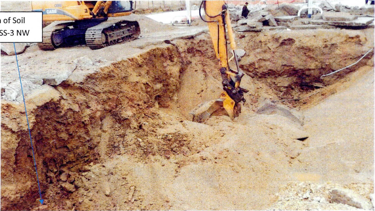
PHOTO 8 – PHOTOGRAPH OF UNDERGROUND STORAGE TANK EXCAVATION FACING SOUTHEAST
