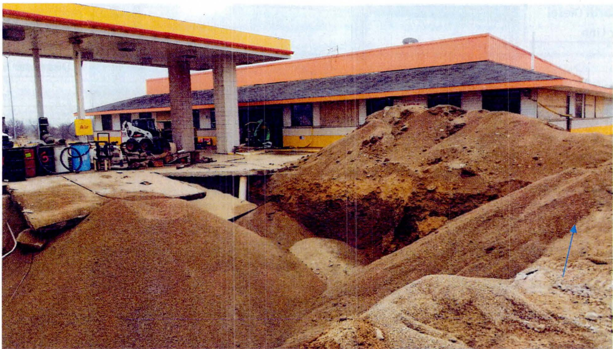
PHOTO 6 – PHOTOGRAPH OF THE SOUTHEASTERN PORTION OF THE EXCAVATION
