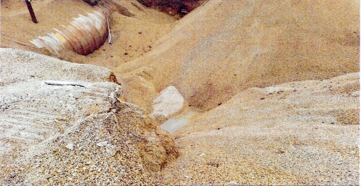
PHOTO 9 – PHOTOGRAPH OF THE WATER IN THE BOTTOM OF THE EXCAVATION
