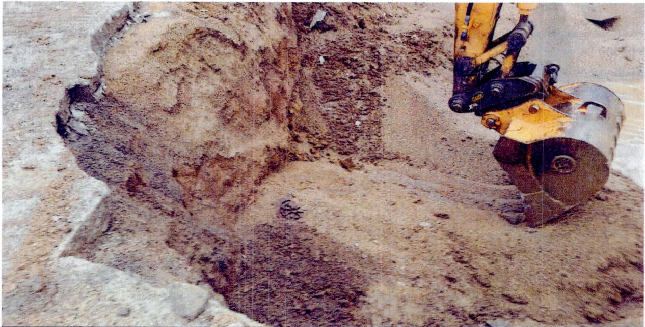
PHOTO 10 – PHOTOGRAPH OF AREA OF SOIL SAMPLE SS-3, NORTHWEST EXCAVATION
