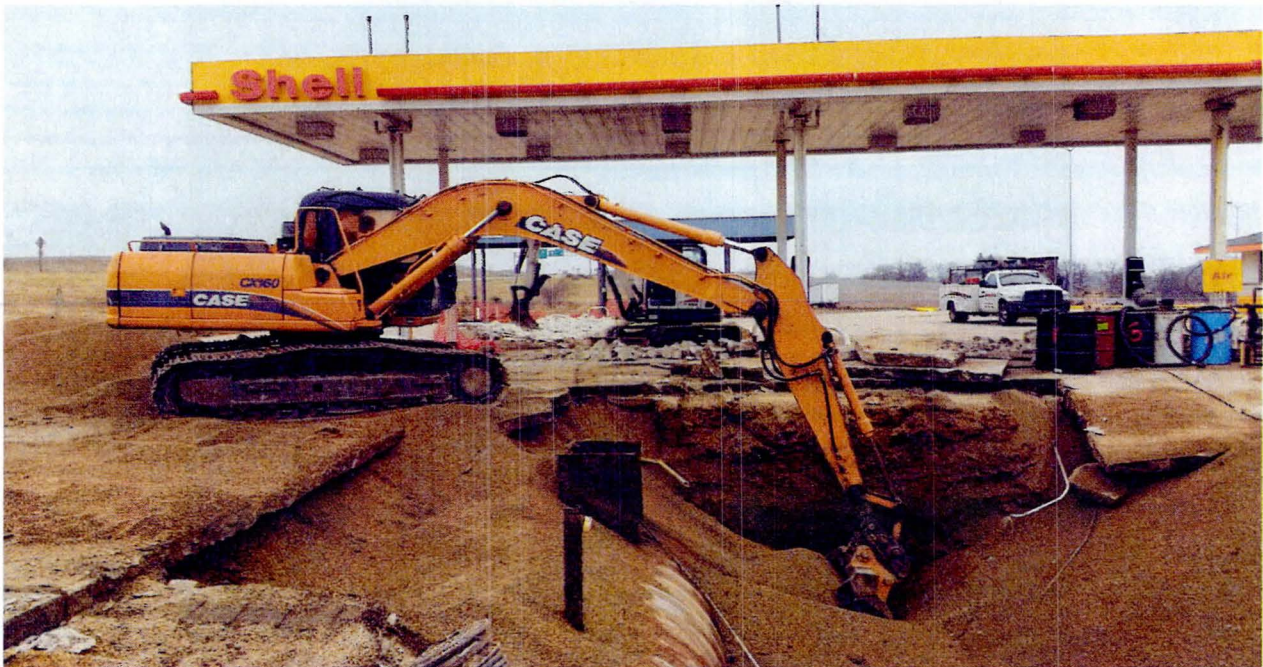
PHOTO 7 - PHOTOGRAPH OF THE NORTHEASTERN PORTION OF THE UNDERGROUND STORAGE TANK EXCAVATION
