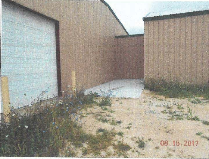
Title: Photo #1: Area of cap to be maintained (looking north/northwest)
