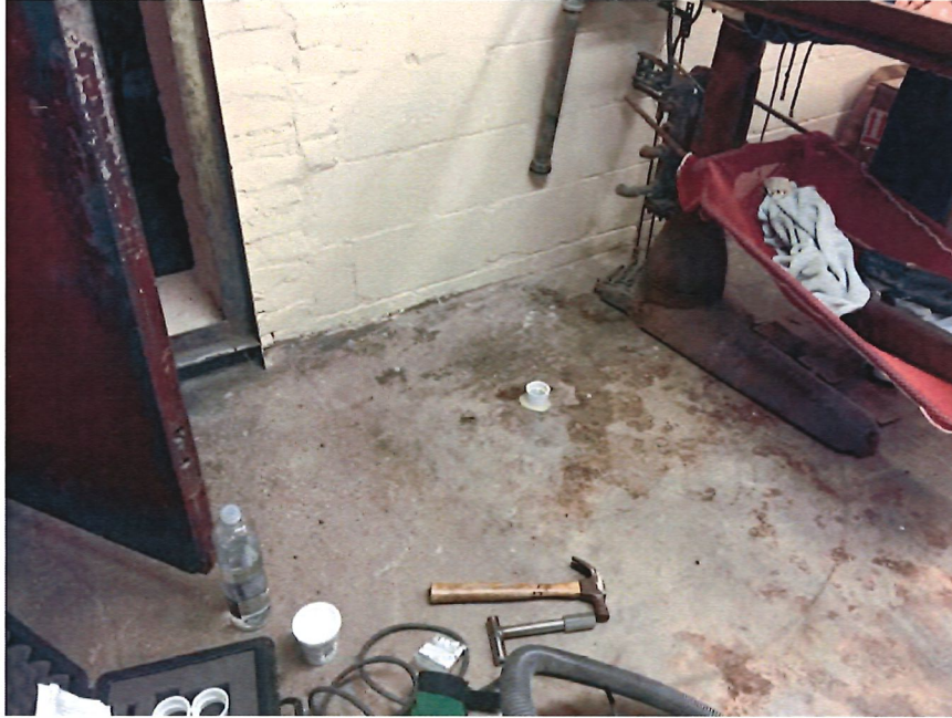
Photo 3: Sub-slab sample point location and water dam test set up.
