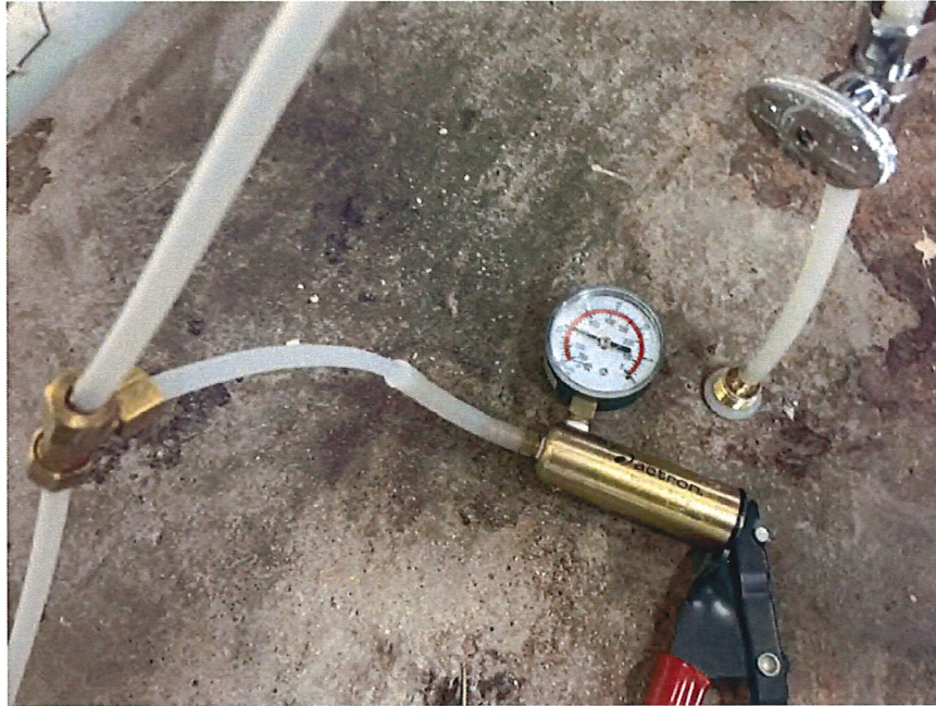
Photo 5: Shut-in test on sub-slab sample train.
