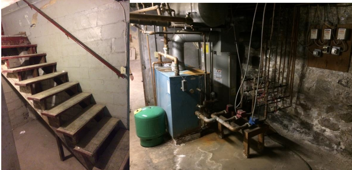
Picture 5 – left: Southern stairway entry
