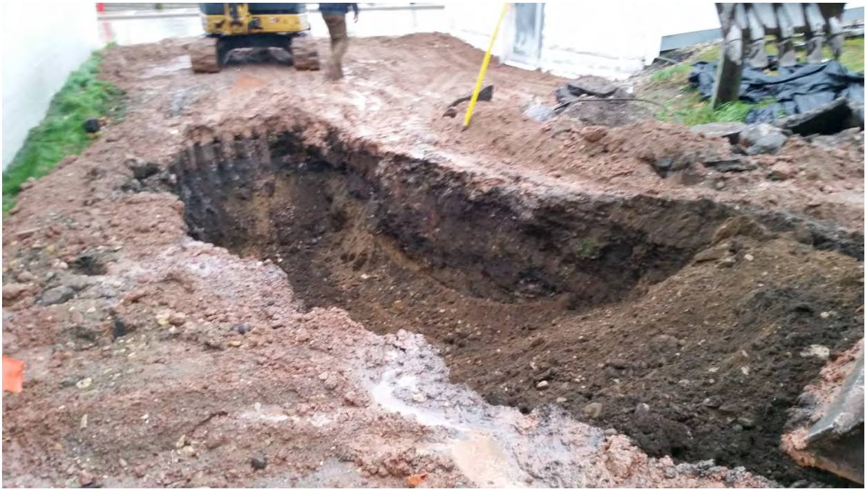
View of excavation
