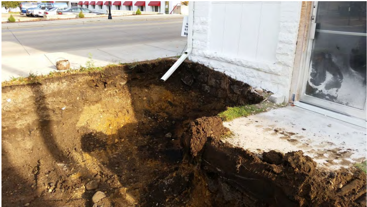
View of excavation area near building
