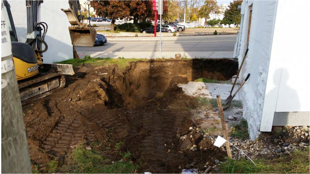
View of excavation looking north
