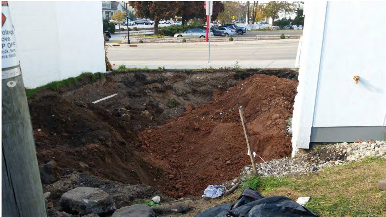
Excavation area, clean fill
