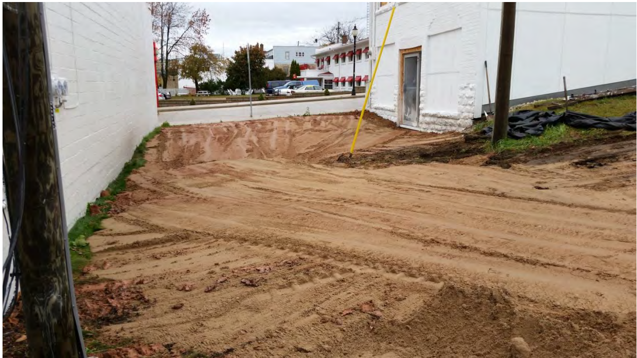
View of completed excavation area looking north
