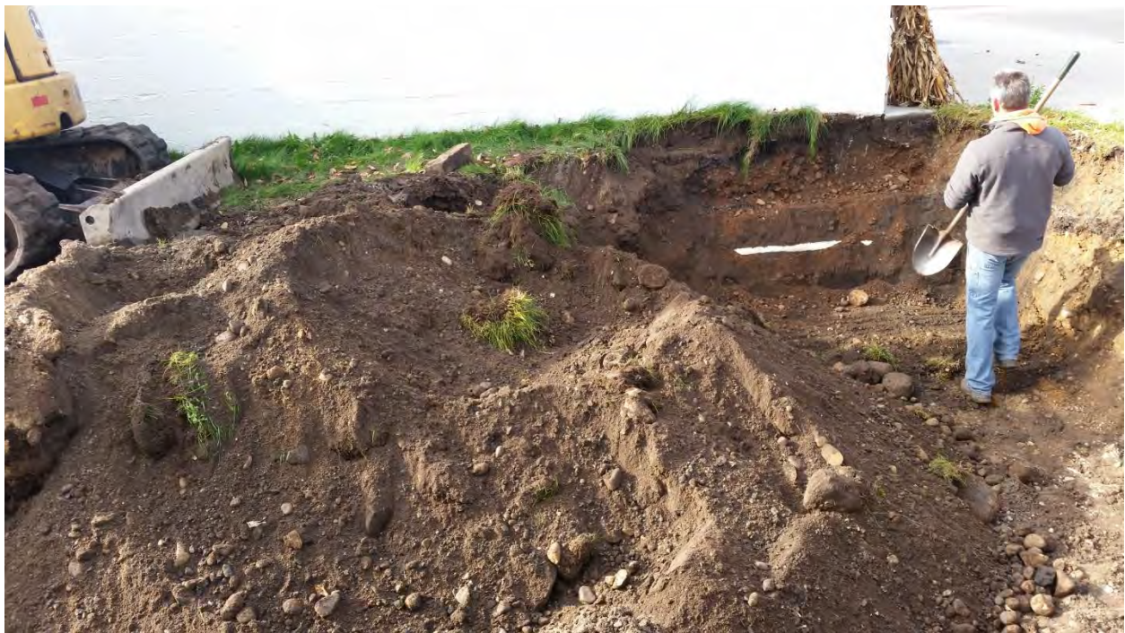
View of excavation area looking west, utility pipe exposed
