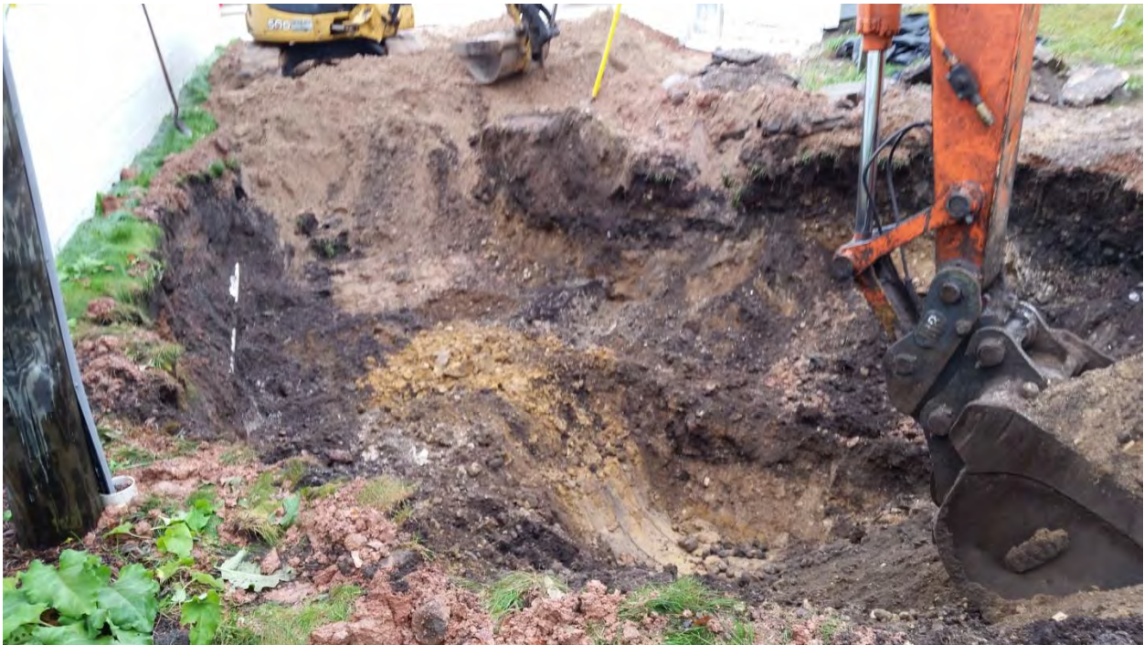
Excavation of hot spot
