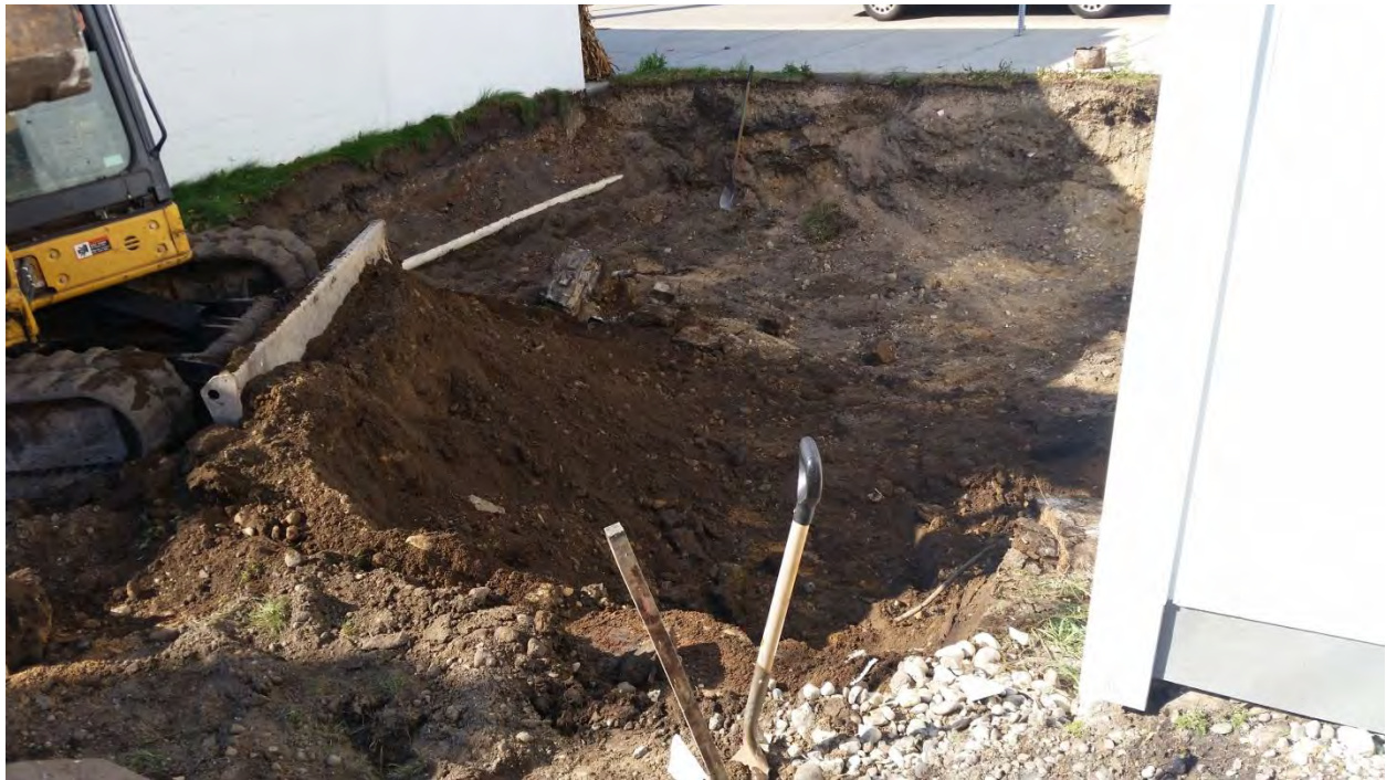
View of excavation area
