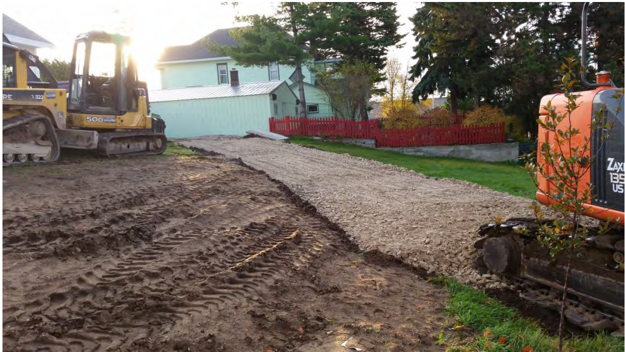
Gravel driveway built to access excavation area
