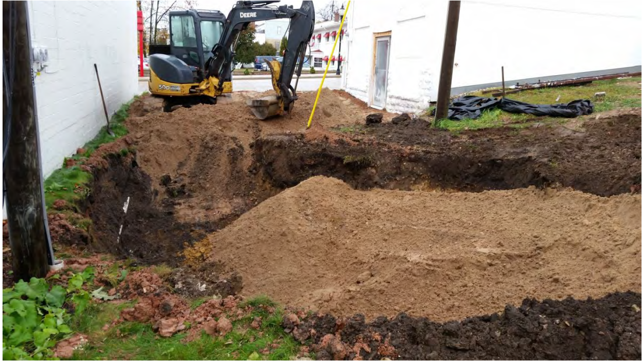
Excavation area, clean fill
