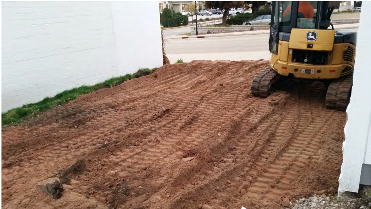
View of compacted fill
