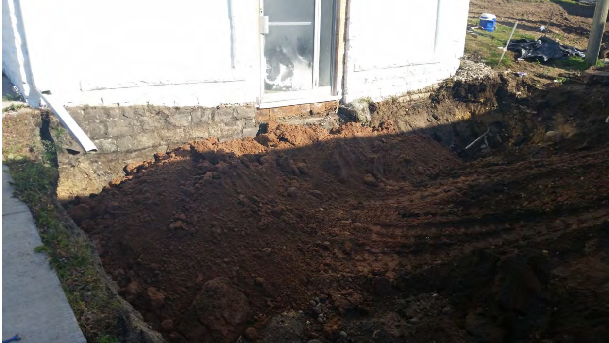
View of excavation looking east, clean fill
