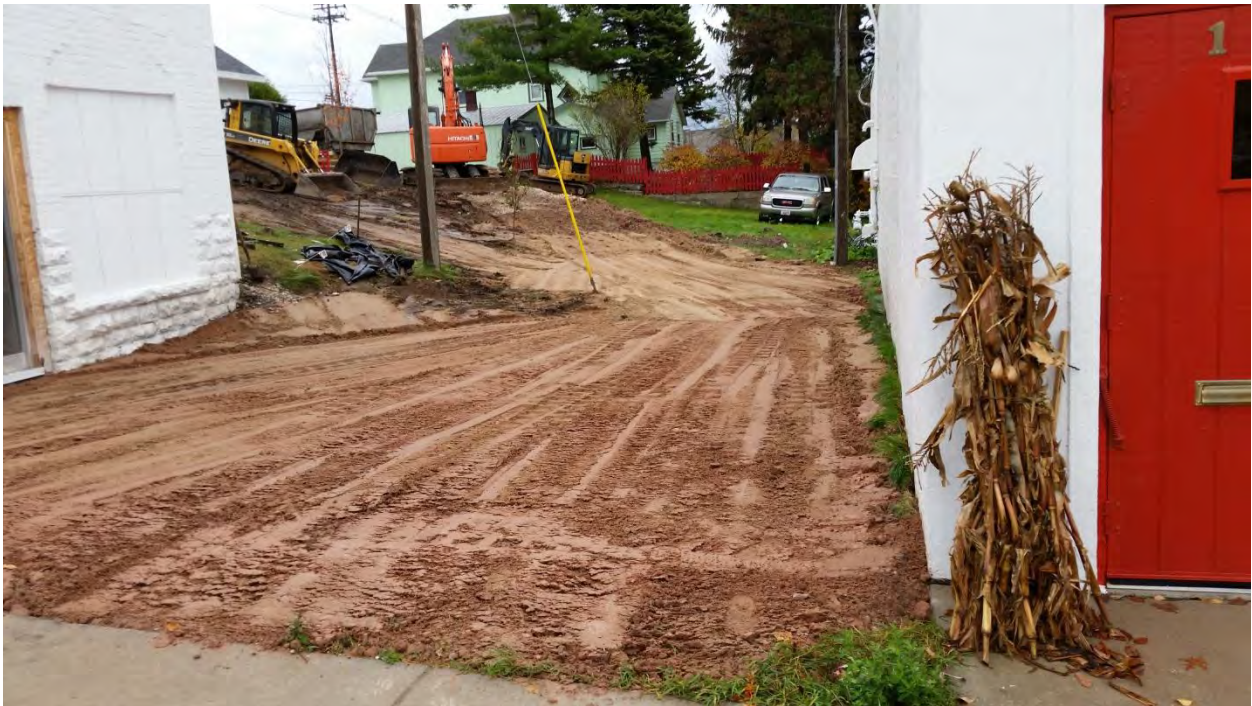
View of completed excavation area looking south
