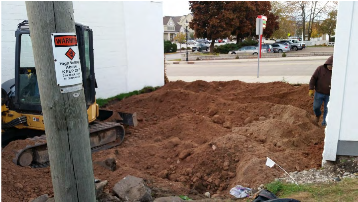
View of clean fill
