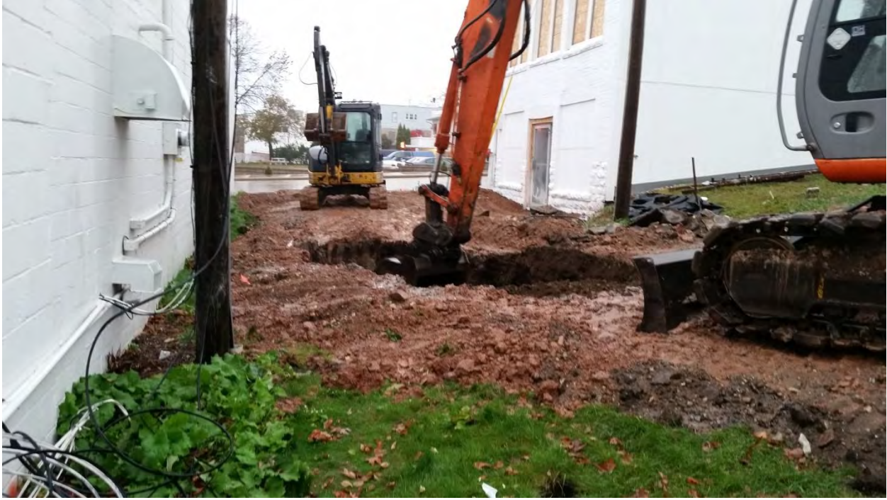
Start of excavation on day 2
