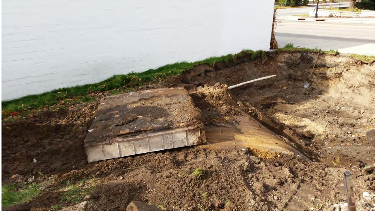
View of concrete slab removed from building
