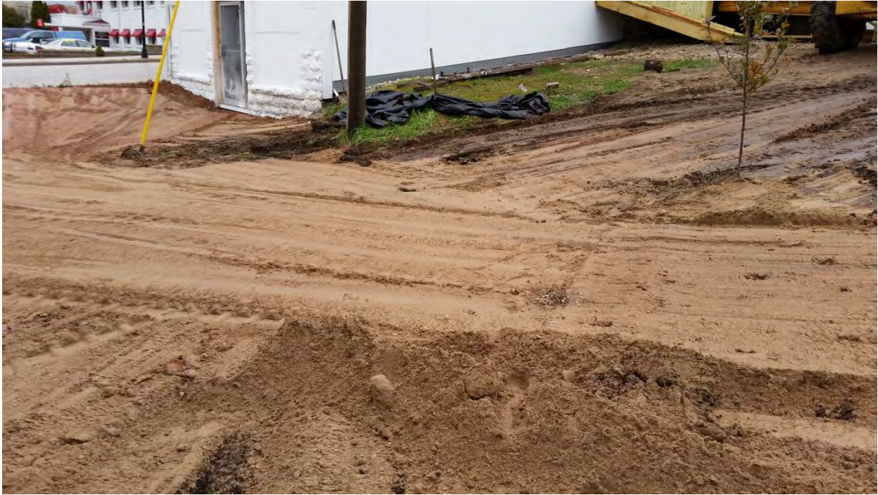
View of completed excavation area looking east
