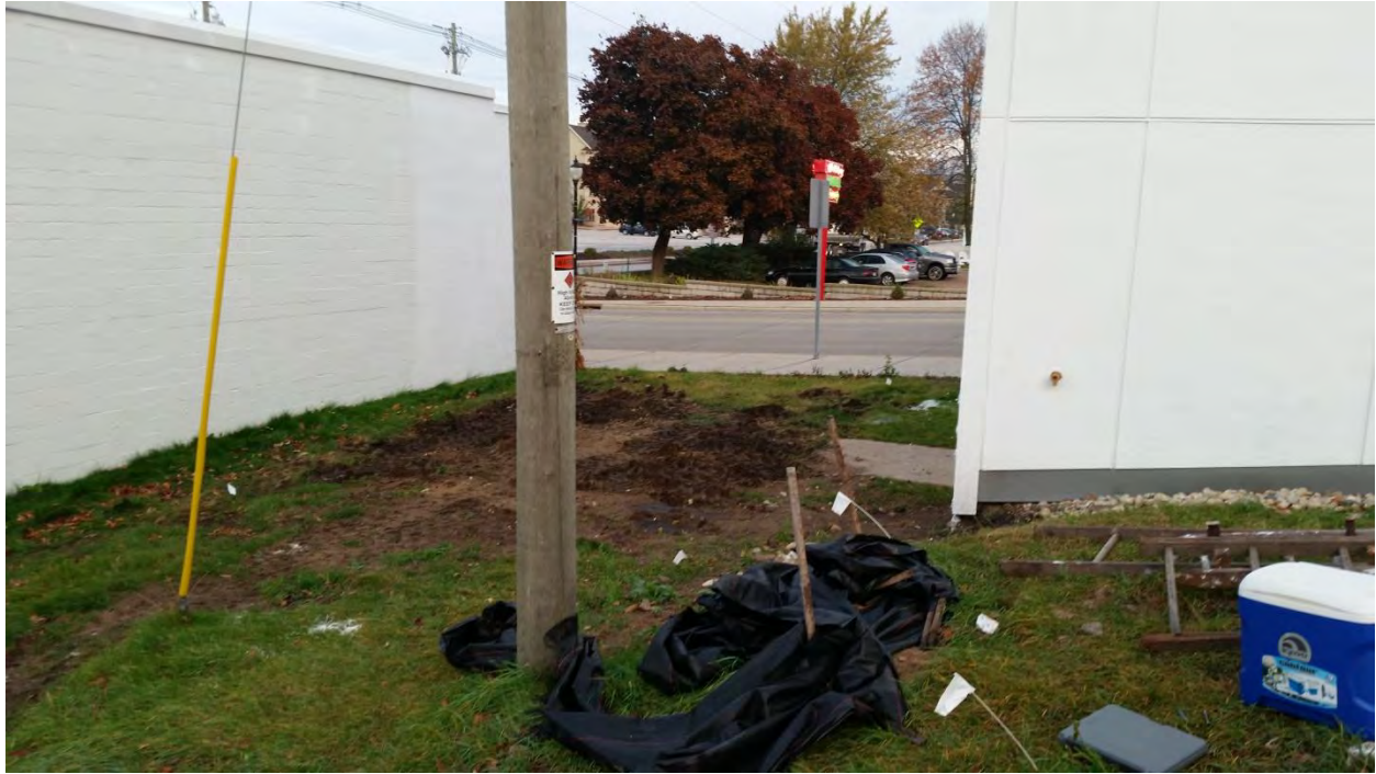
Excavation area, 7 South 2nd Ave, Sturgeon Bay, WI
