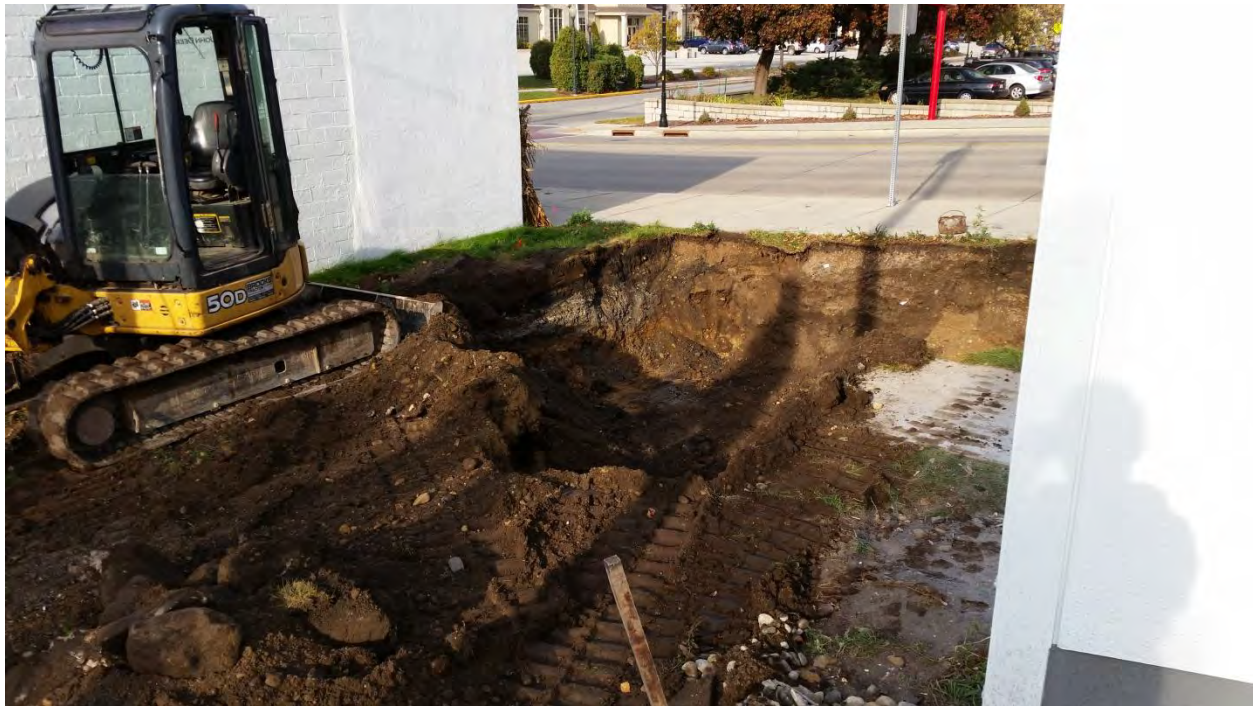
View of excavation area
