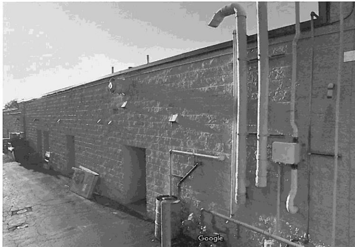
11. Protective barrier of asphalt in parking lot. MW-1 and PZ-1 outside the back door of Krystal Kleeners.
