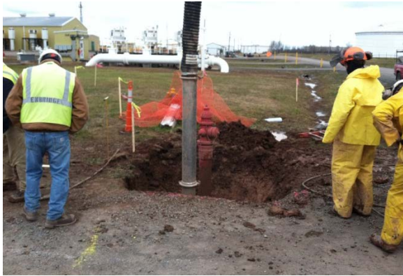
Photo 1: Fire hydrant removal excavation on 11/1/2012. The photo was taken facing east.
