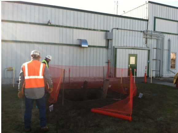
Photo 4: Office water valve removal excavation. The photo was taken facing west.
