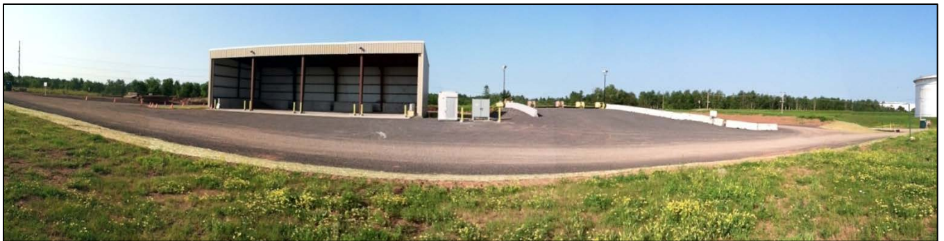
Photo 3: The permanent SMA Facility. The contaminated solid soil stockpile building is on the left and the contaminated slurry soil ramp is on the right. The photo was taken facing west on July 29, 2013.
