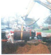
UST / AST Removal
