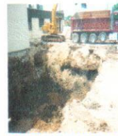
CONTAMINATED SOIL EXCAVATIONS
