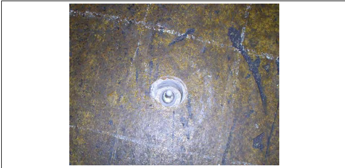
Typical Vapor Pin sub-slab sampling point
