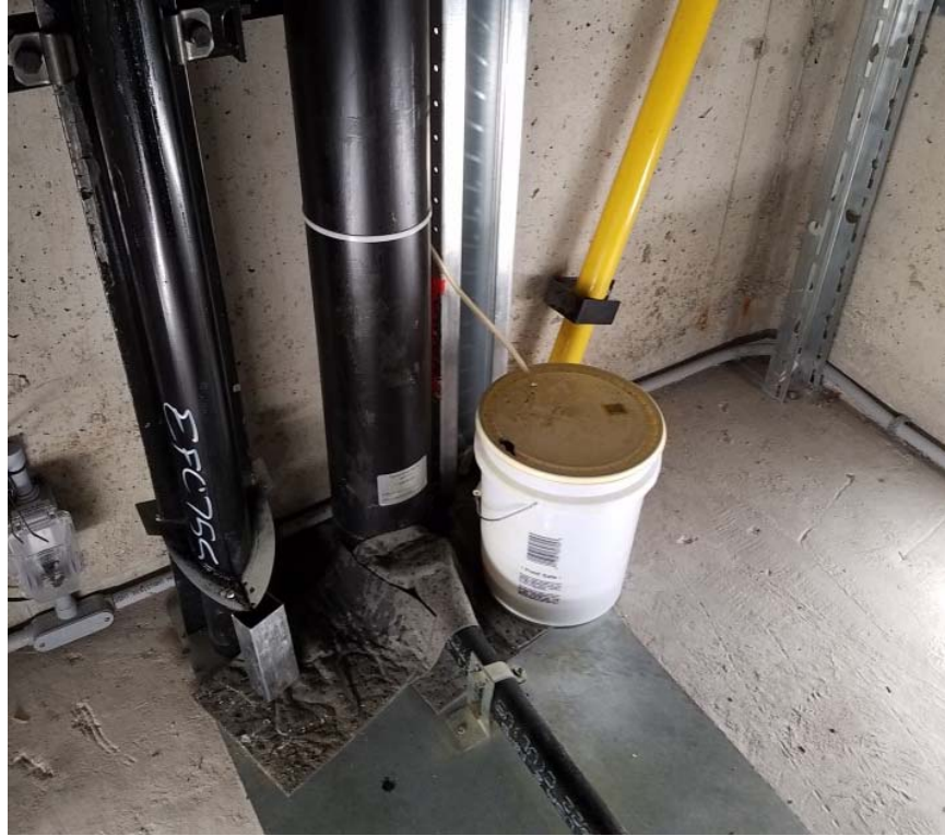
Photograph 1: Typical construction of elevator pit
