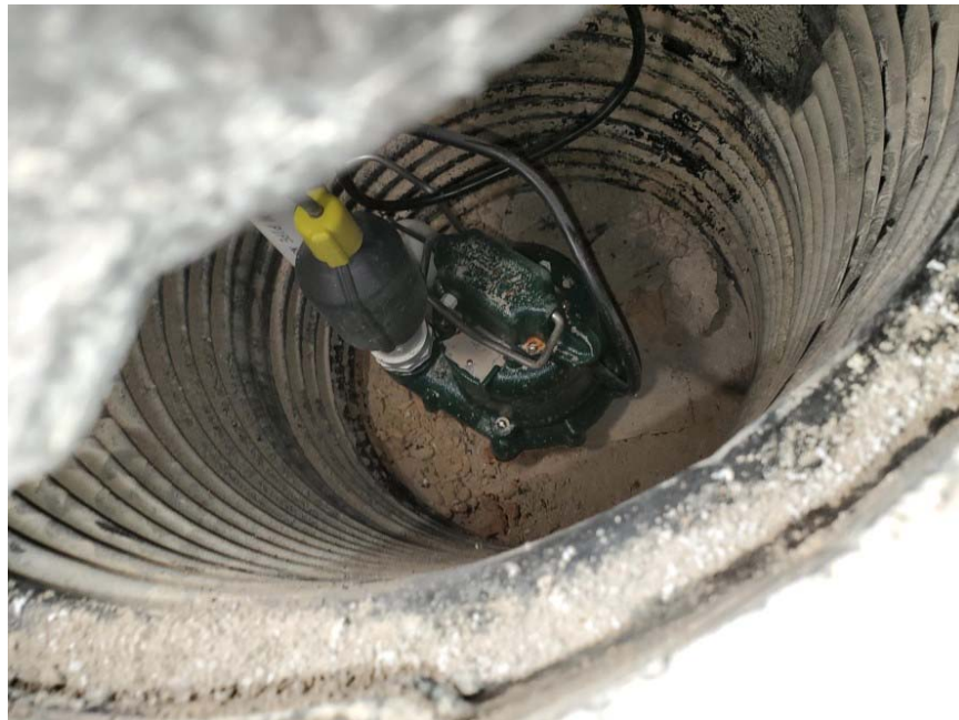
Photograph 8: View of the sump bottom
