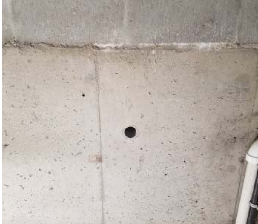
Photograph 5: Pipe penetration through west wall of elevator pit
