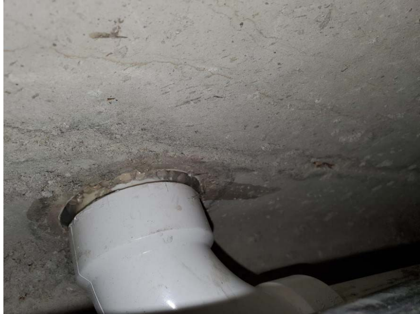
Photograph 7: Silicon caulk around sump discharge piping penetration
