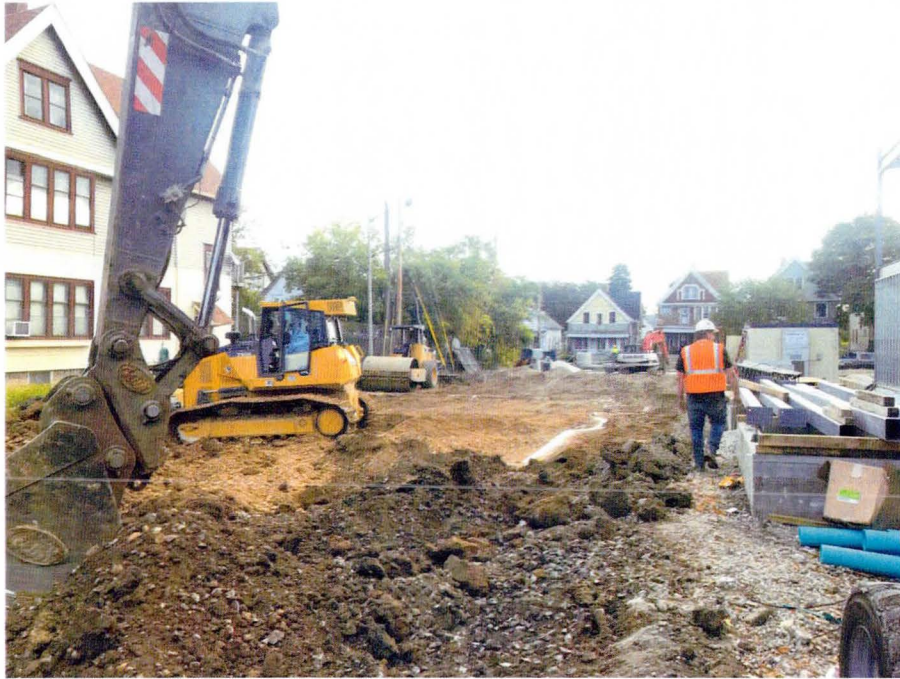
Photo 5: Parking lot subgrade removal in progress in northwest portion of Site on October 4, 2017. View looking to east.
