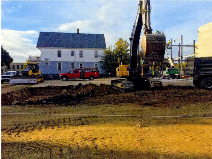
Photo 3: Parking lot subgrade removal (including area for pervious pavers and underlying storm water retention) in progress in northeast portion of Site on October 3, 2017. View looking to south.
