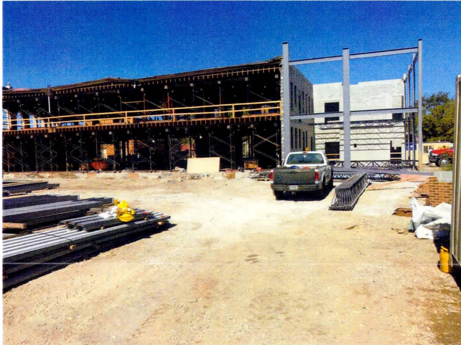
Photo 9: First 18 inches of clay placed for green space soil cover system in south portion of Site (currently used for outdoor staging) on October 4, 2017. View looking to north.
