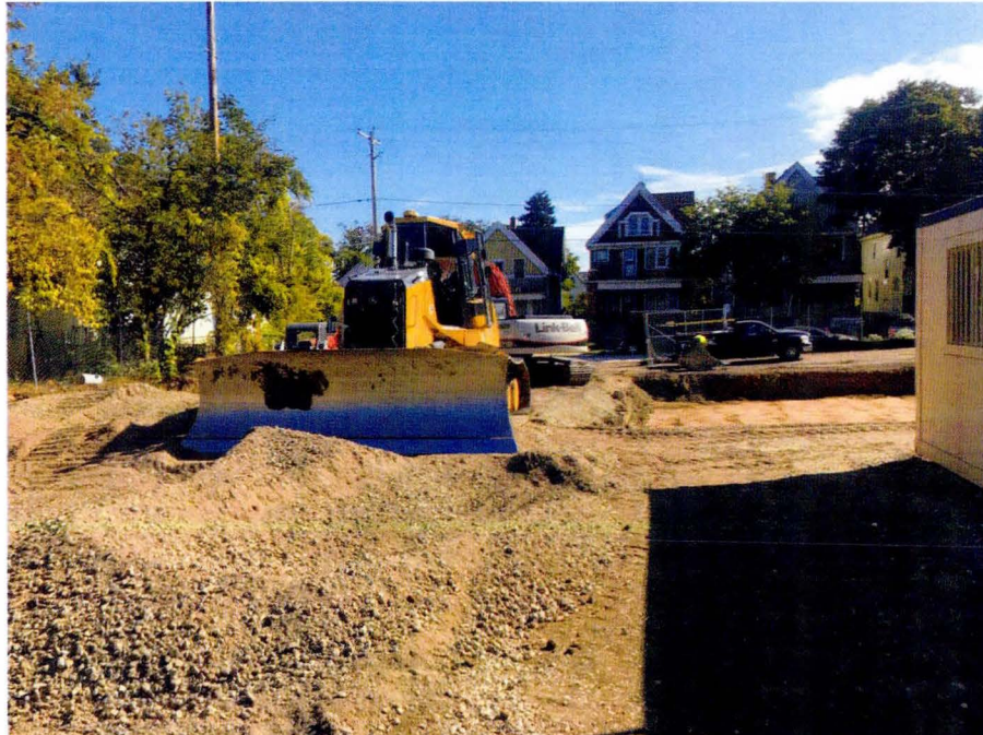
Photo 6: Gravel subgrade being placed in north portion of Site for new asphalt parking lot on October 4, 2017. View looking to east.
