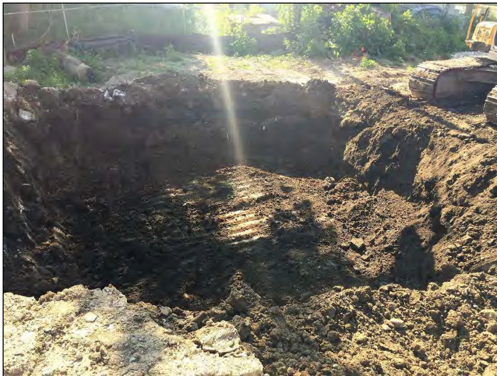
Photo 2: Remedial excavation around GP-7/GP-7R area. View looking east.
