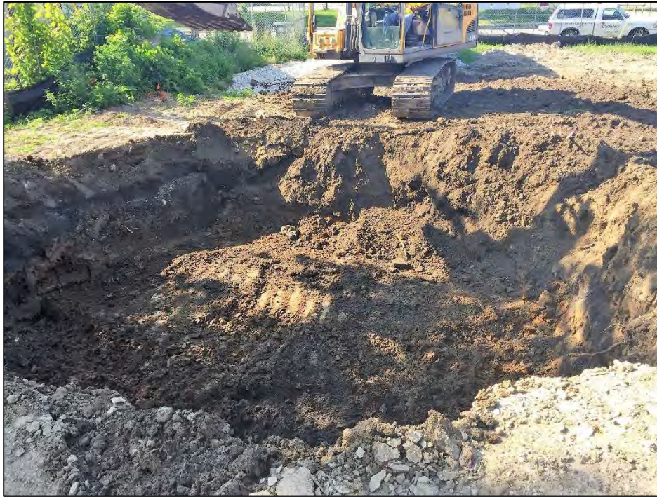
Photo 1: Remedial excavation around GP-7/GP-7R area. View looking southeast.
