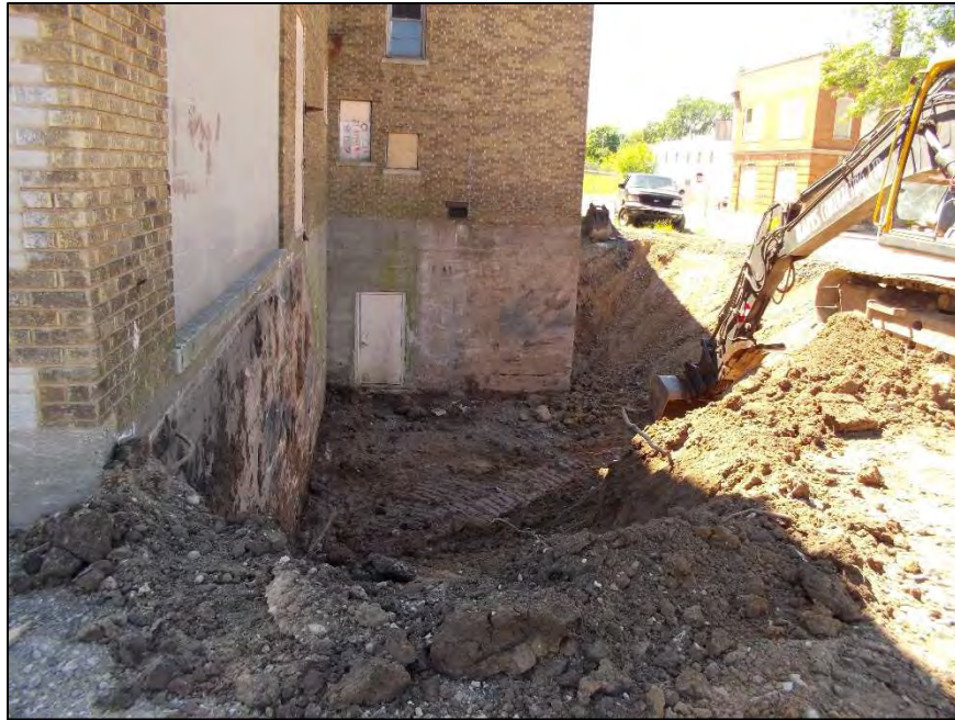
Photo 1: Excavation in northern portion of new basement area on June 6, 2017. View looking west.
