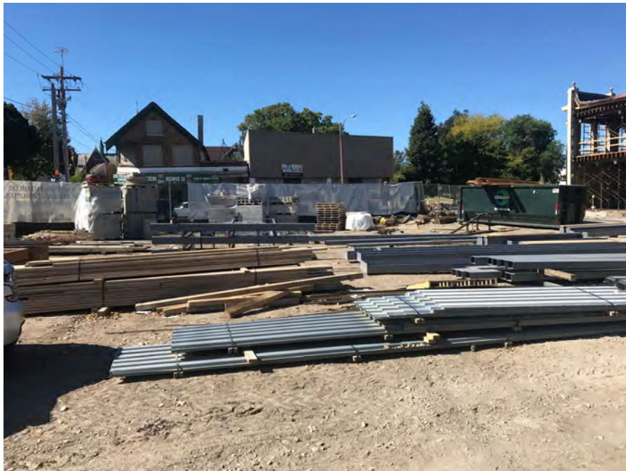
Photo 8: First 18 inches of clay placed for green space soil cover system in south portion of Site (currently used for outdoor staging) on October 4, 2017. View looking to west.
