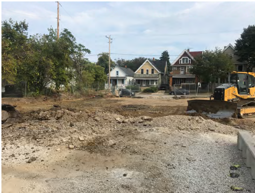
Photo 2: Parking lot subgrade removal in progress in northeast portion of Site on October 2, 2017. View looking to east.
