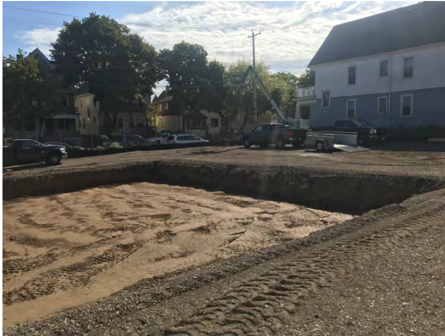
Photo 7: Gravel subgrade placed and compacted in northeast portion of Site for new asphalt parking lot on October 4, 2017. View looking to southeast.
