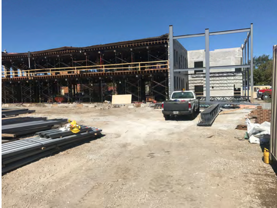
Photo 9: First 18 inches of clay placed for green space soil cover system in south portion of Site (currently used for outdoor staging) on October 4, 2017. View looking to north.
