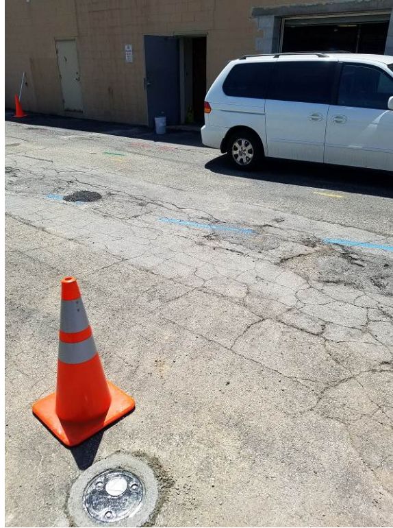
Photo 7: Looking southeast from alleyway behind dry cleaner unit at monitoring well MW-3 (June 1, 2017). The monitoring well MW-4 location is visible in the background adjacent to the building and traffic cone.
