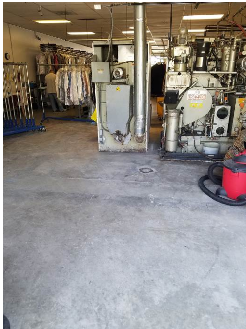
Photo 4: Looking south from north end of dry cleaner unit at back side of dry cleaning machines (June 1, 2017). Monitoring well MW-2 is visible in floor in front of the dry cleaning machines.
