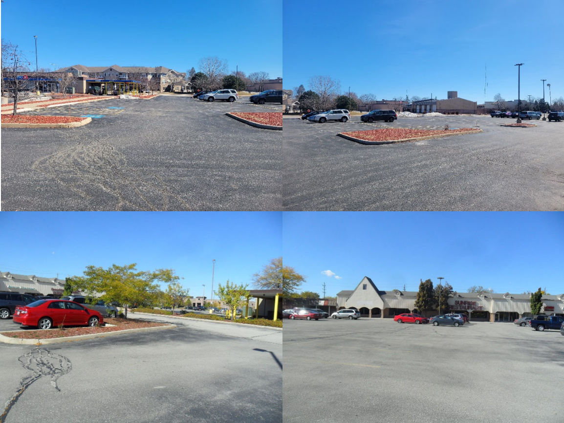
IMAGES OF ASPHALT PAVEMENT WITHIN EASTERN PARKING LOT IMPLEMENTED AS ENGINEERED BARRIER; CLEAN SOIL LANDSCAPE ISLANDS (LIMITED) WITHIN PARKING LOT ALSO IMPLEMENTED AS ENGINEERED BARRIER
