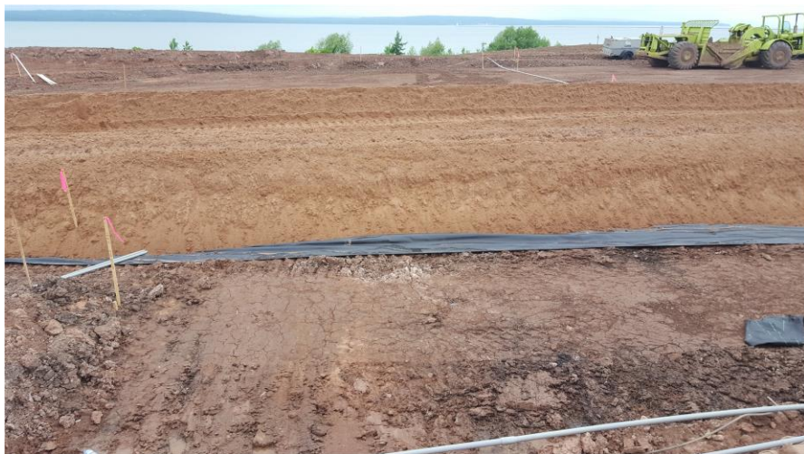
Location of excavation after grading looking north.
