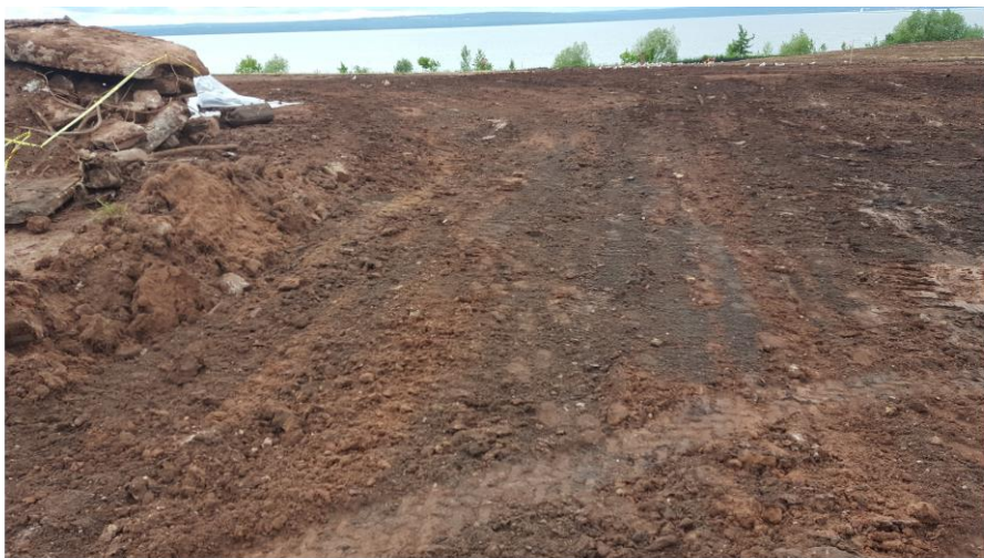
Location of excavation of petroleum impacted material looking north.
