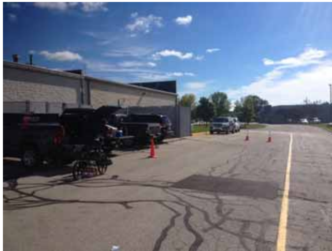
Photo No. 2 showing the clearance of underground utilities in the rear of the Bright Cleaners tenant space using ground penetrating radar, view to the northeast.
