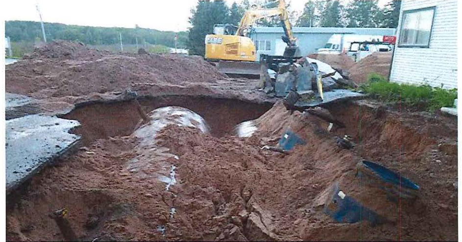
View of tank basin facing west.
