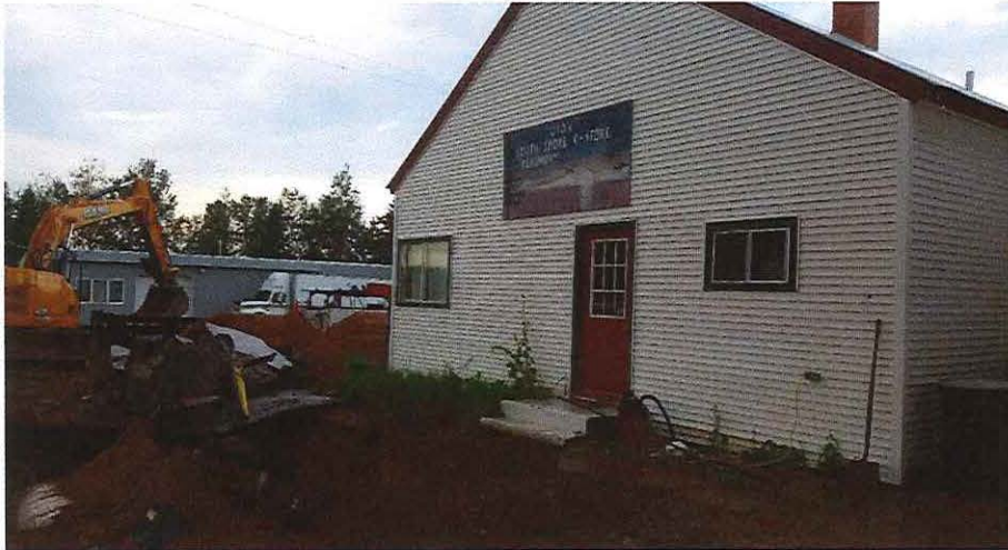
View of tank basin and C-Store Laundromat building facing northwest.
