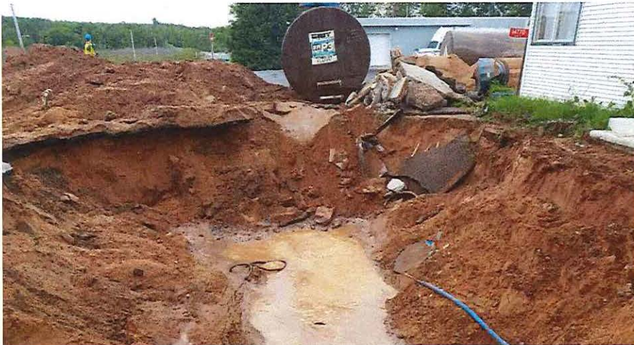
View of groundwater filling excavation.
