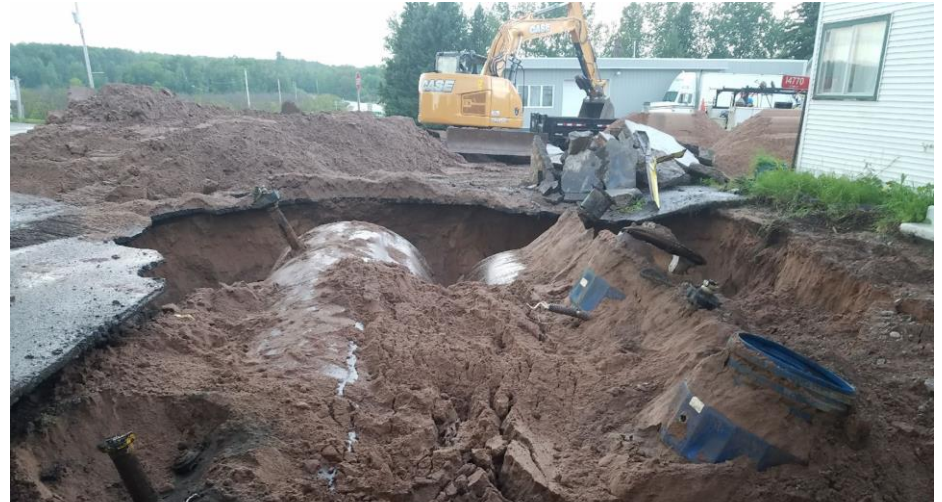
View of tank basin facing west.
