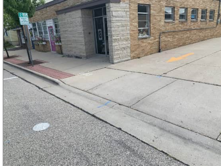
Title: West side of building (facing N/NE)
