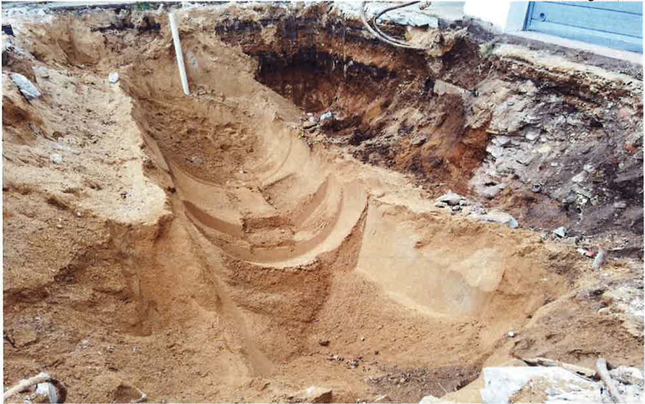
PHOTOGRAPH OF THE BOTTOM ON THE EXCAVATION BENEATH THE 10,000-GALLON TANK
