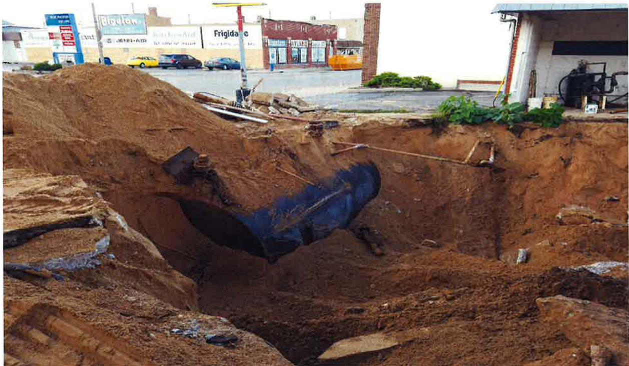
PHOTOGRAPH OF SOIL BENEATH THE NORTHERNMOST 8000-GALLON TANK
