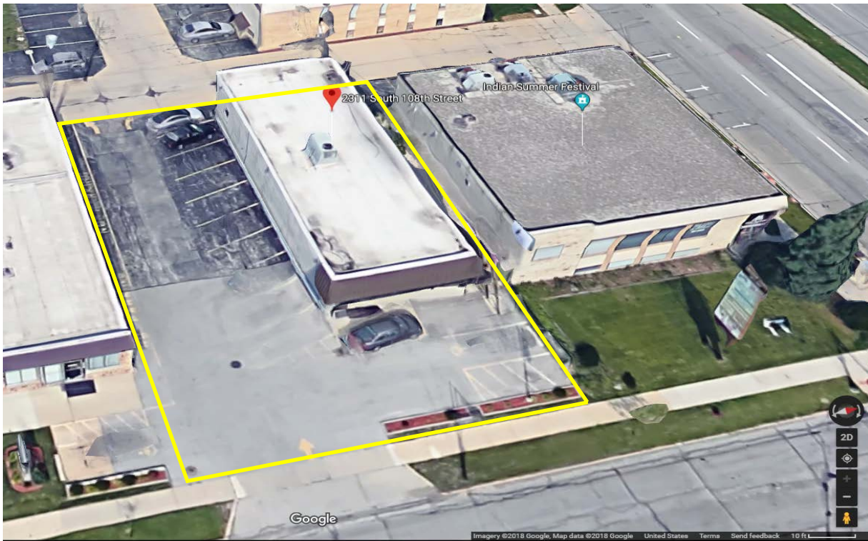
Subject Property – Facing northwest, aerial view showing property extents
