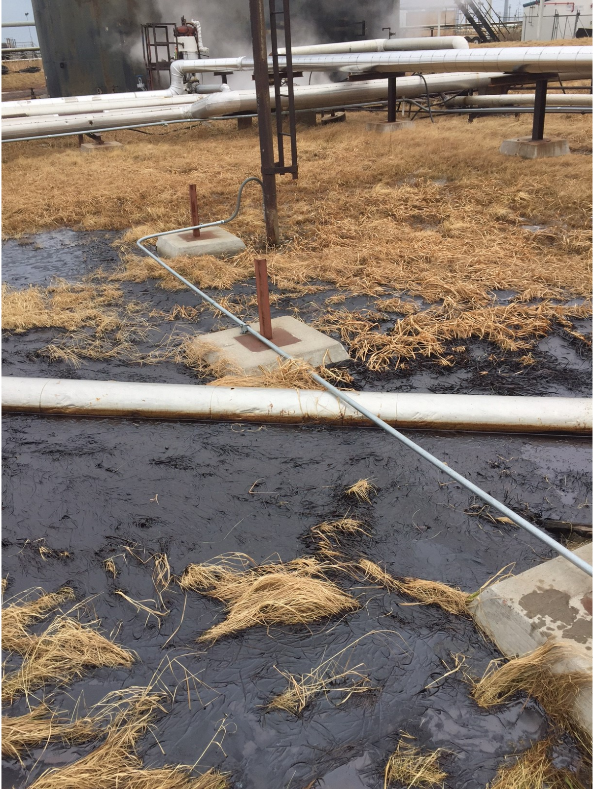
Photo 3: Looking southeast at the middle of the release.
