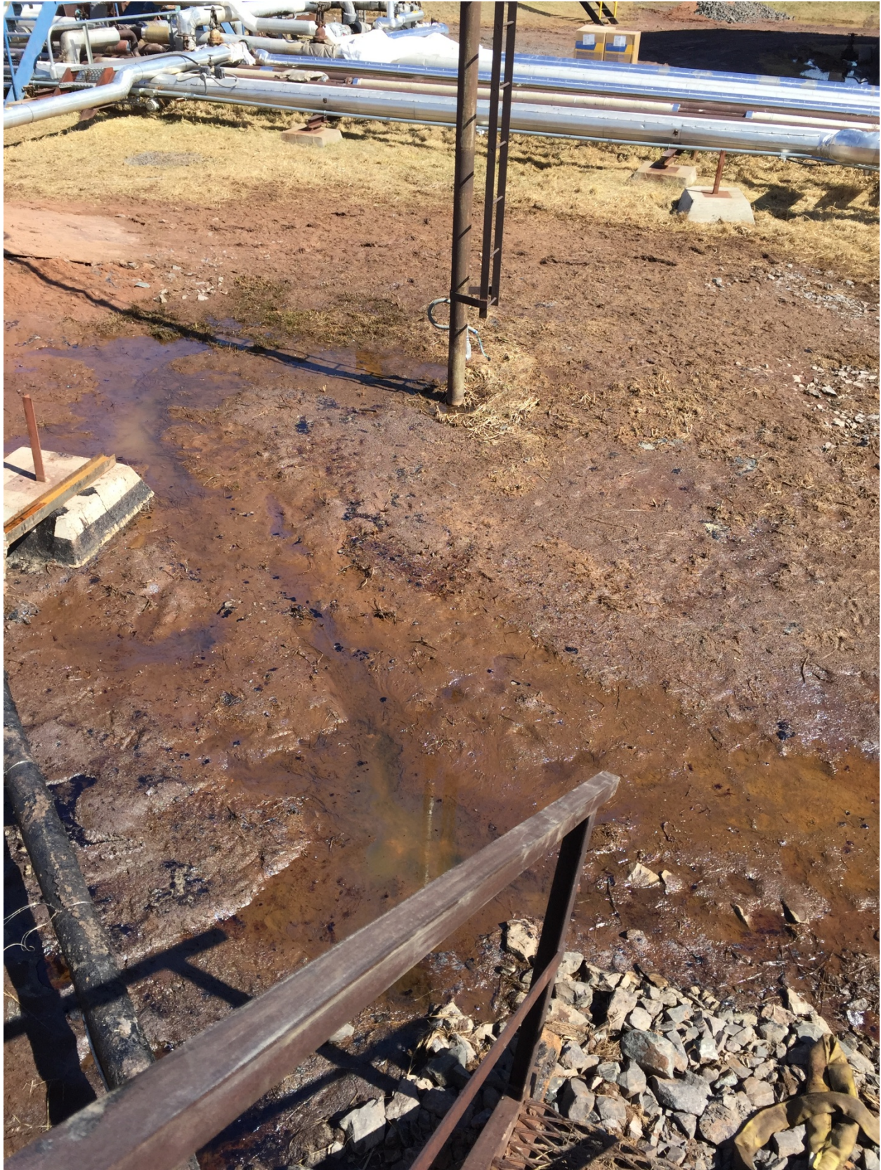
Photo 7: Looking east at the release site after the initial excavation.
