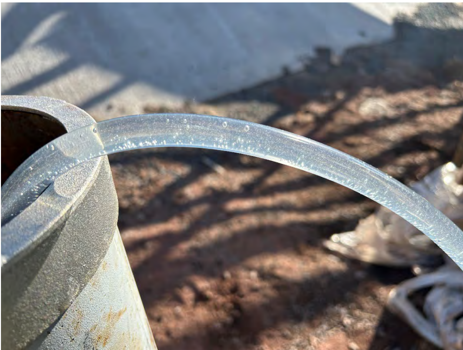
Photo 6: IW-1 development water clearing up after pumping, photo facing east; photo taken on 3/12/2024.
